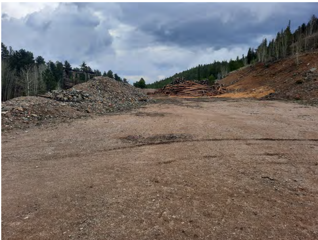
Figure 15. Landing area above creek. Note piles and ore bin on left. Logs will be removed from site in late fall of 2023. Spoils from excavation will be distributed across toe of slope on right.
