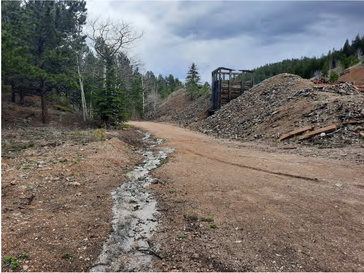
Figure 9. Sherwood Creek percolating through overburden along road. New alignment would follow existing road. Waste rock piles and historic ore bin in background. May 18, 2023.
