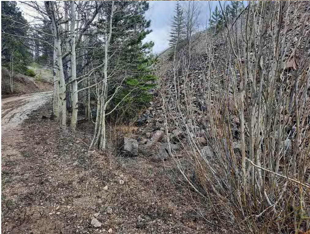
Figures 11, 12. Dry portions of Sherwood Creek along base of tailing pile, May 18, 2023. This low swale will receive some on-site fill, while maintaining the existing woody vegetation. The new stream alignment will be to the left of the current depression, on a portion of the existing access road.
