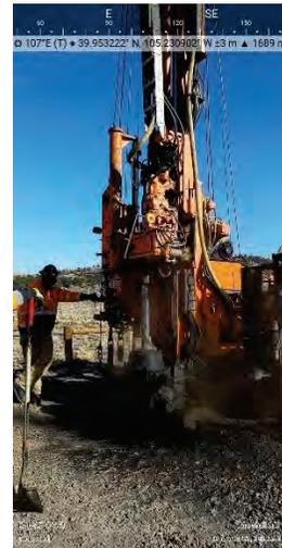
PHOTOGRAPH 16 02-24-2022 MM-26 Drilling through coal
