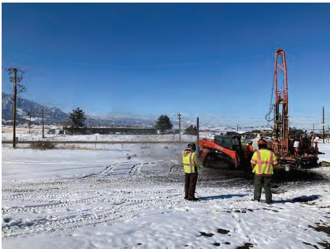
PHOTOGRAPH 9 02-24-2022 MM-06 Drilling through coal.
