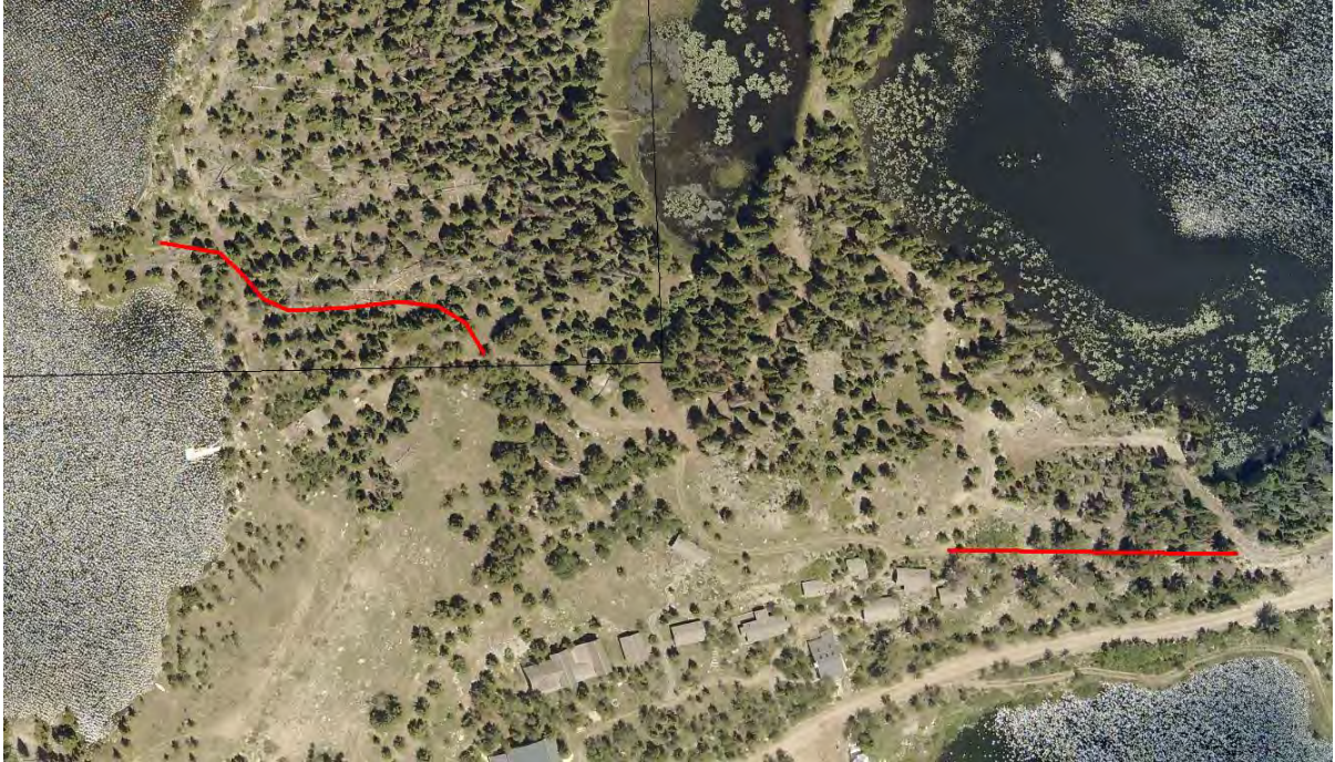
Figure 3. New road segments, constructed without permit.
