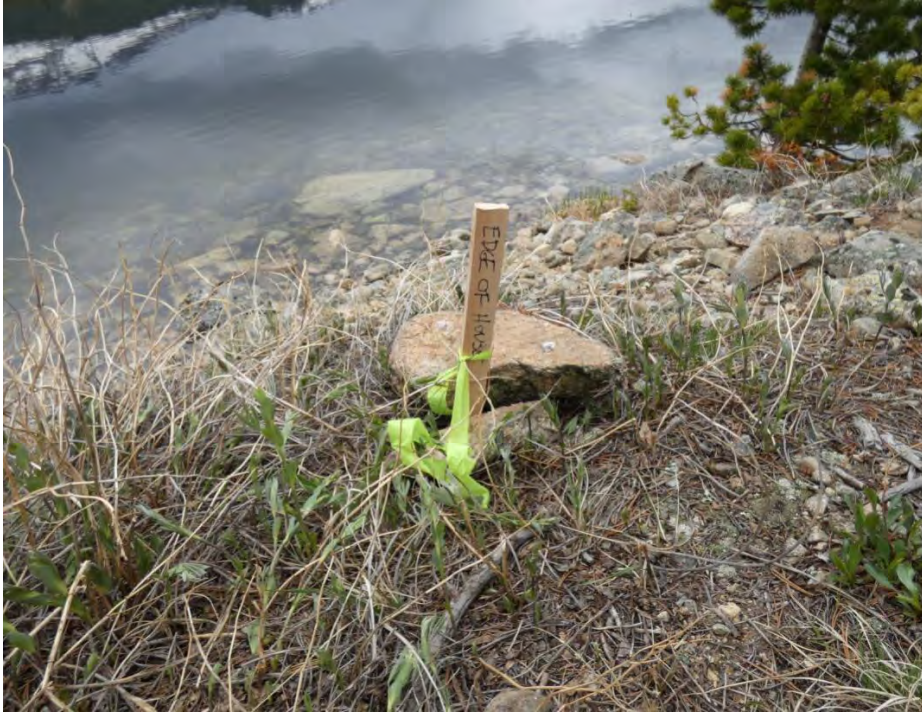
Figure 1A -- A construction stake at the site -- "Edge of House"
