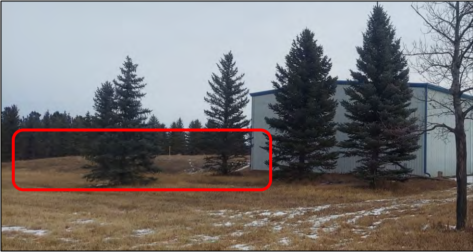
Figure 9: Photo of existing barn with raised septic system area indicated in red.
