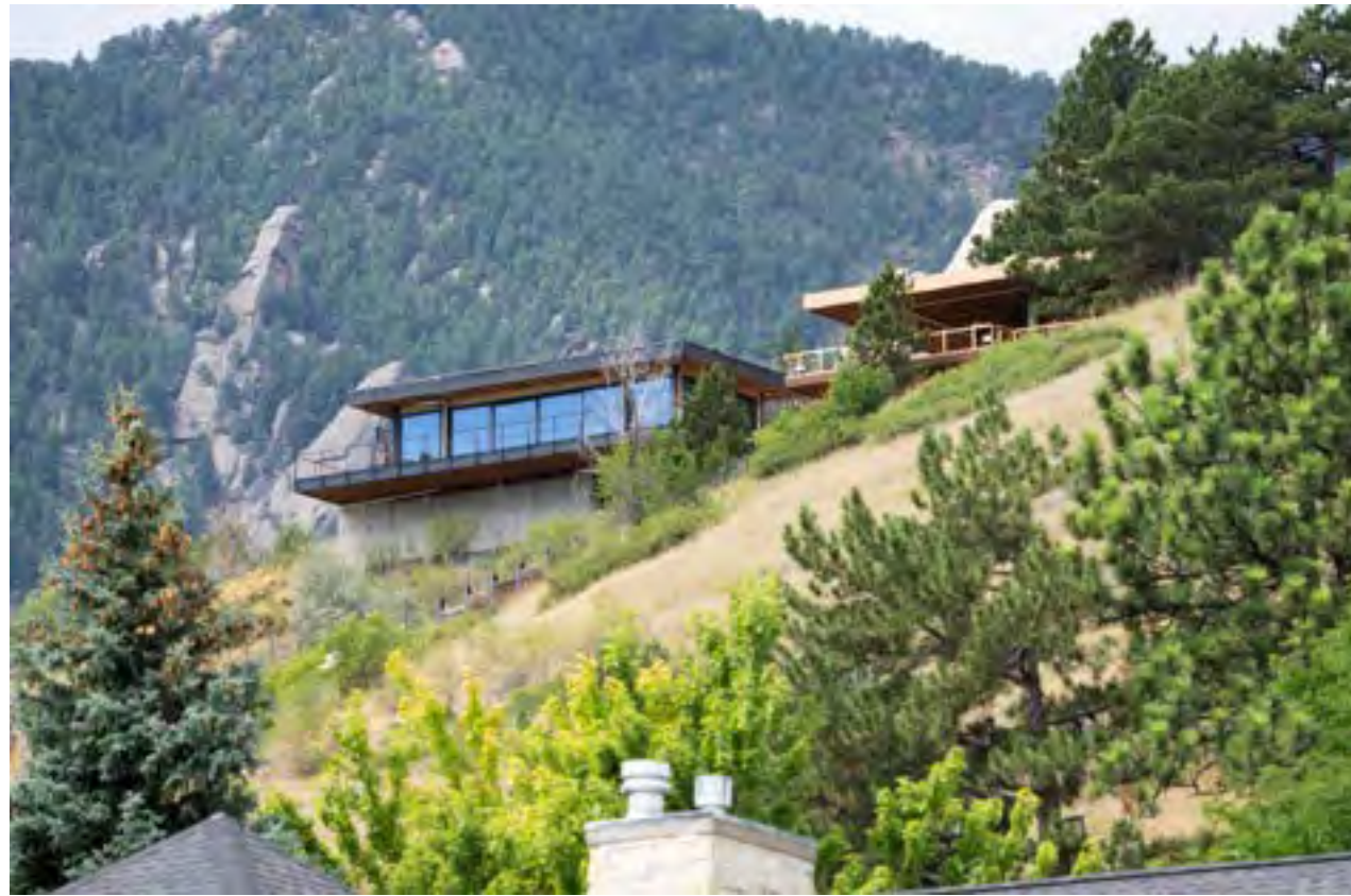
1 NE View from King Ave - Existing
