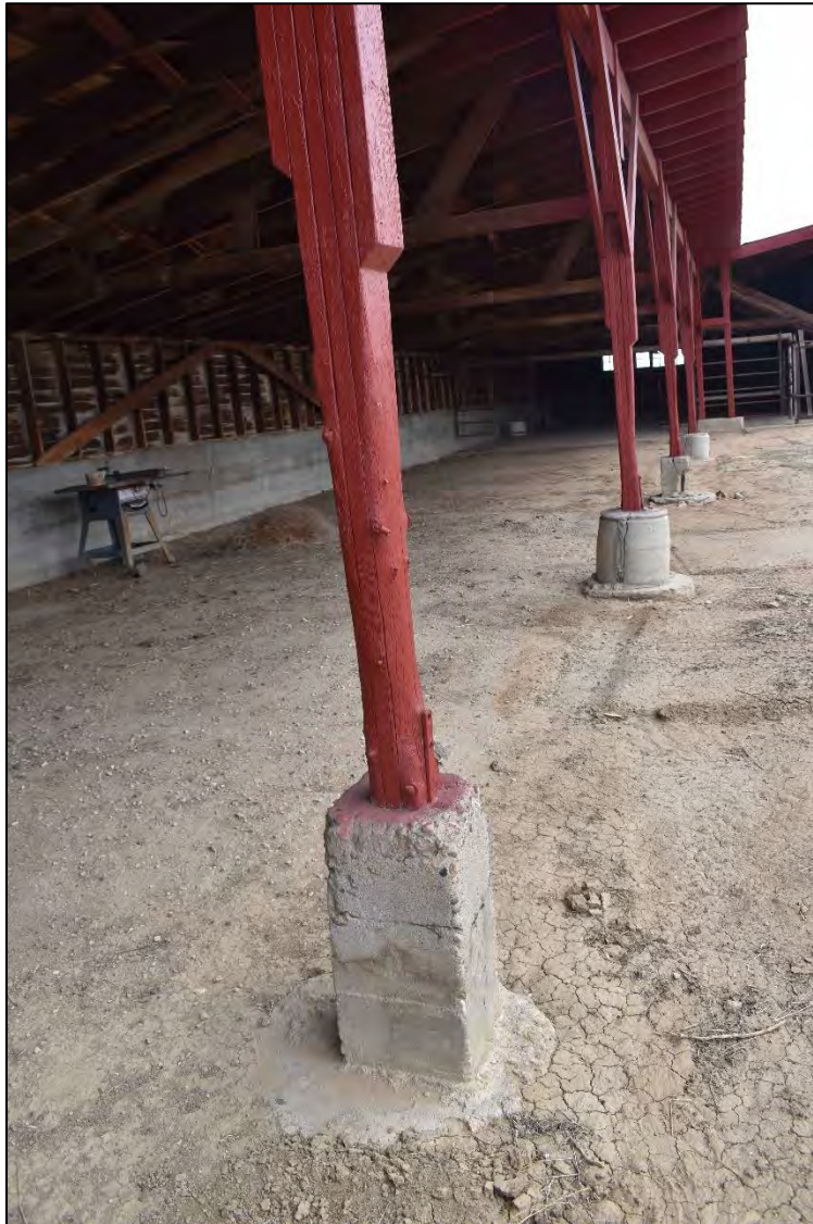
34 of 59. North loafing shed (Resource H), interior, showing post worn by cattle rubbing. View east-northeast.
