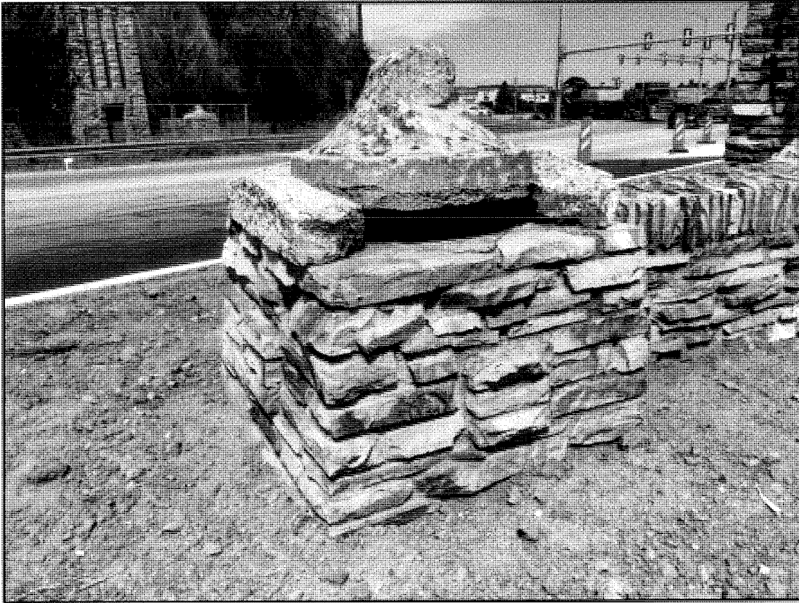
5BL.432, southern pillar, west side pier with decorative cast concrete element, looking NNE.
