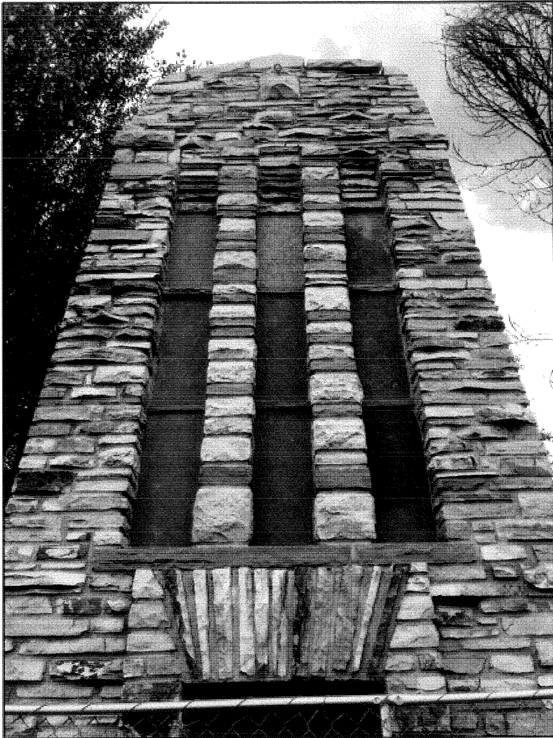
5BL.432, south side of northern gateway pillar, looking north and showing the ashlar stonework and tall, narrow window panels that are now sealed with wood.
