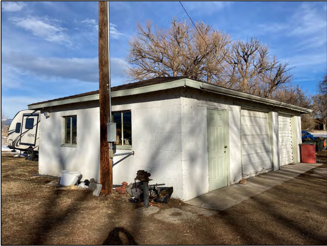
Shop/Garage – southeast elevation – February 9, 2022
