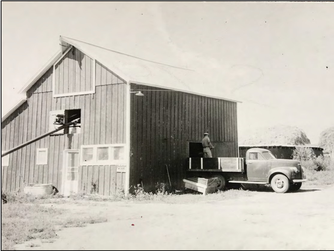
Barn - northeast elevation - Boulder County Assessor photo - circa 1949
