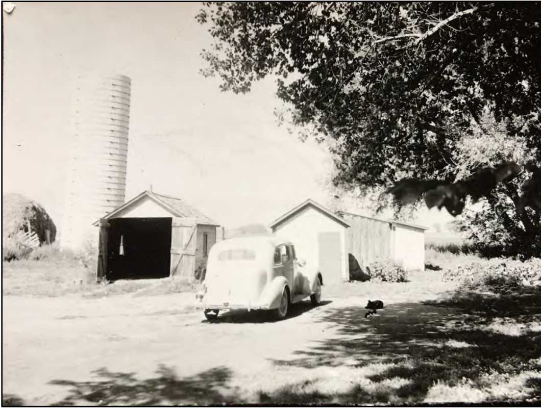
left to right - silo (no longer present), garage (no longer present), shed (no longer present), chicken house (behind shed), privy ( behind shed, no longer present) – looking west Boulder County Assessor photo - circa 1949
