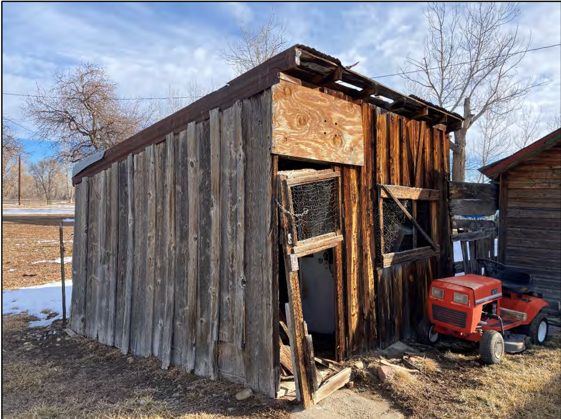
Chicken house – southwest elevation – February 9, 2022
