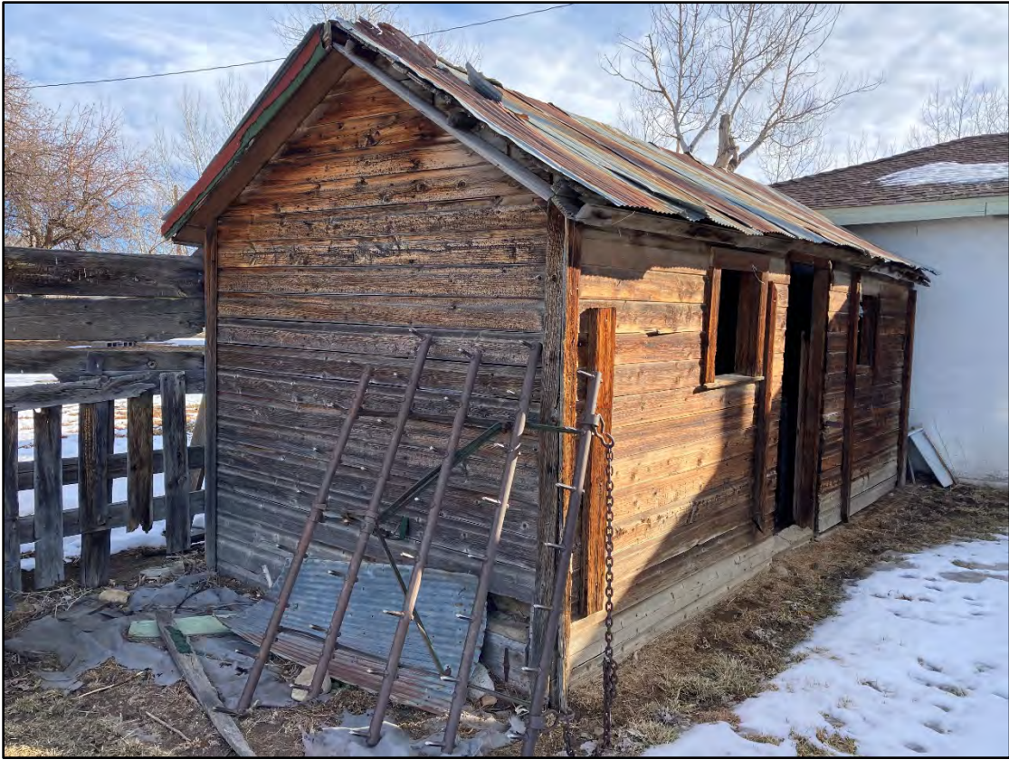
Shed – southwest elevation – February 9, 2022
