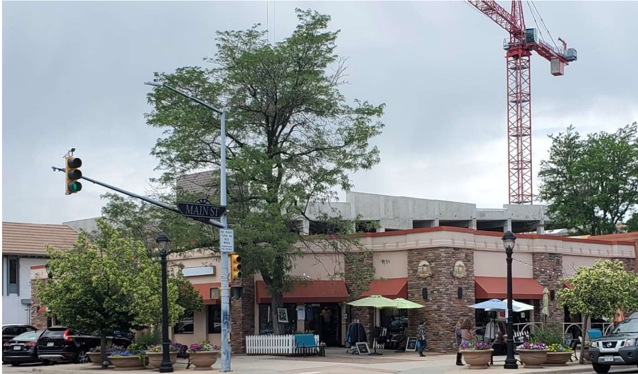
View of garage construction from southeast (5 th and Main)
