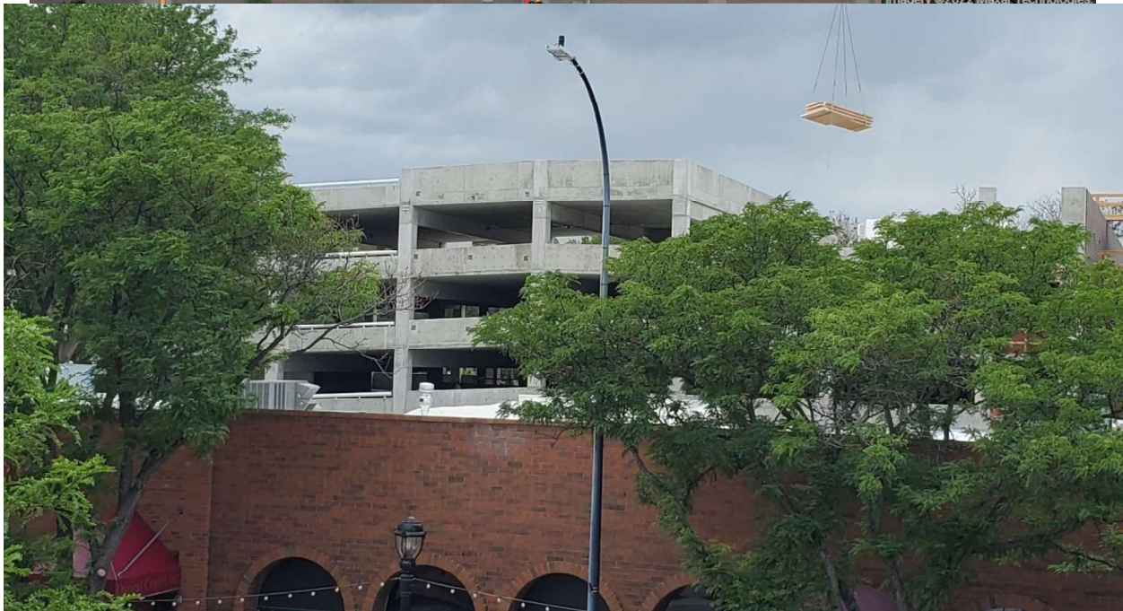
View of garage construction from the northeast (Roost rooftop)
