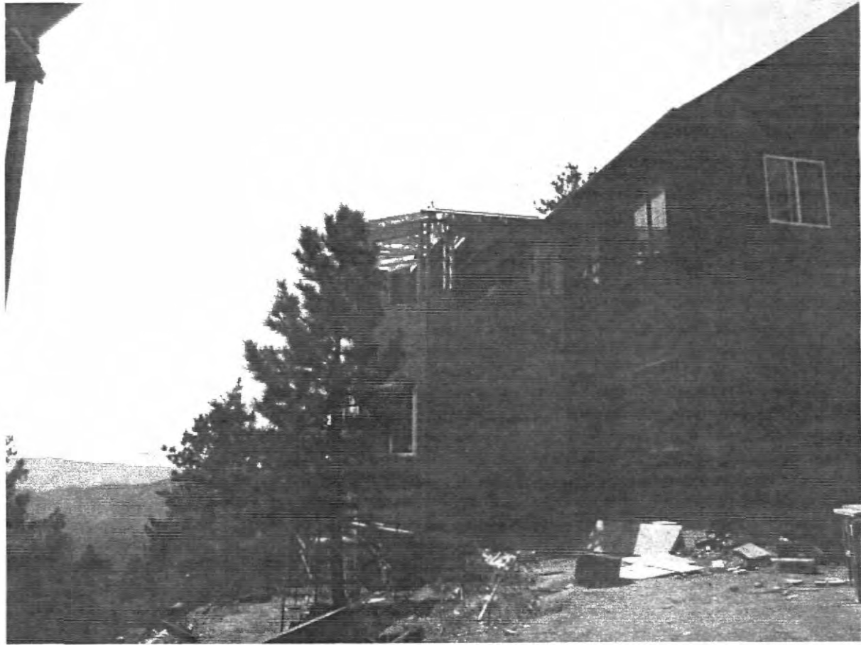
EAST SIDE OF DWELLING - CURRENT CONSTRUCTION
