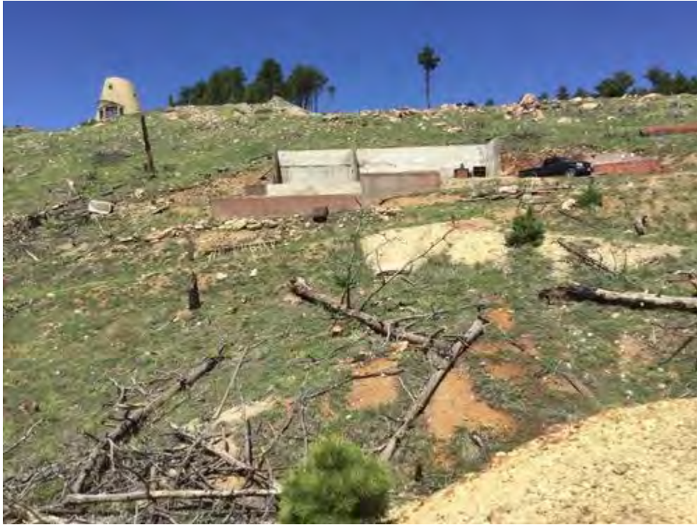
Upper Sweet Home: Looking uphill from MP-01 at foundation with residence in background
