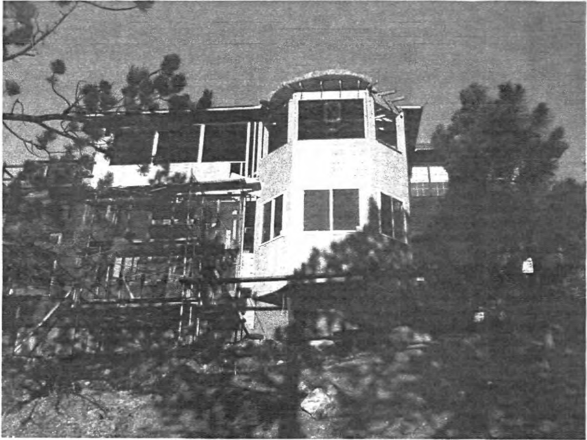
EAST SIDE OF DWELLING - CURRENT CONSTRUCTION
