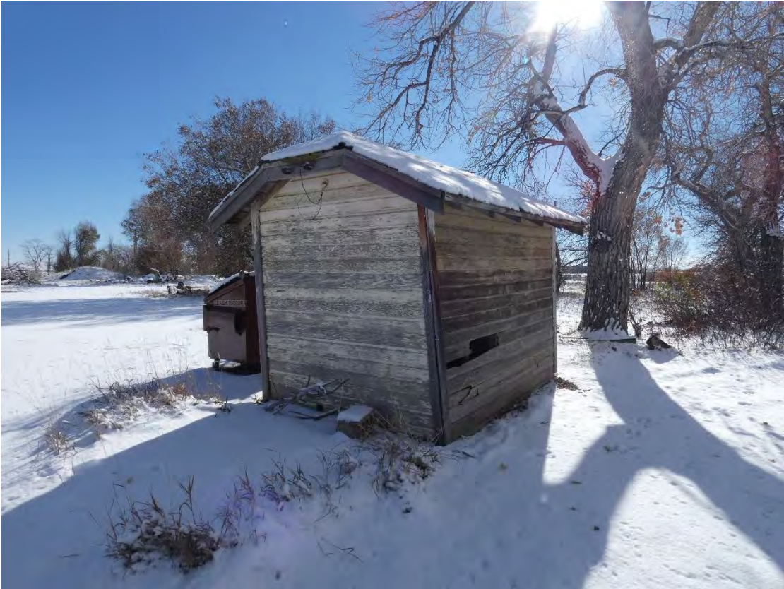
Wood Shed Northwest Elevation
