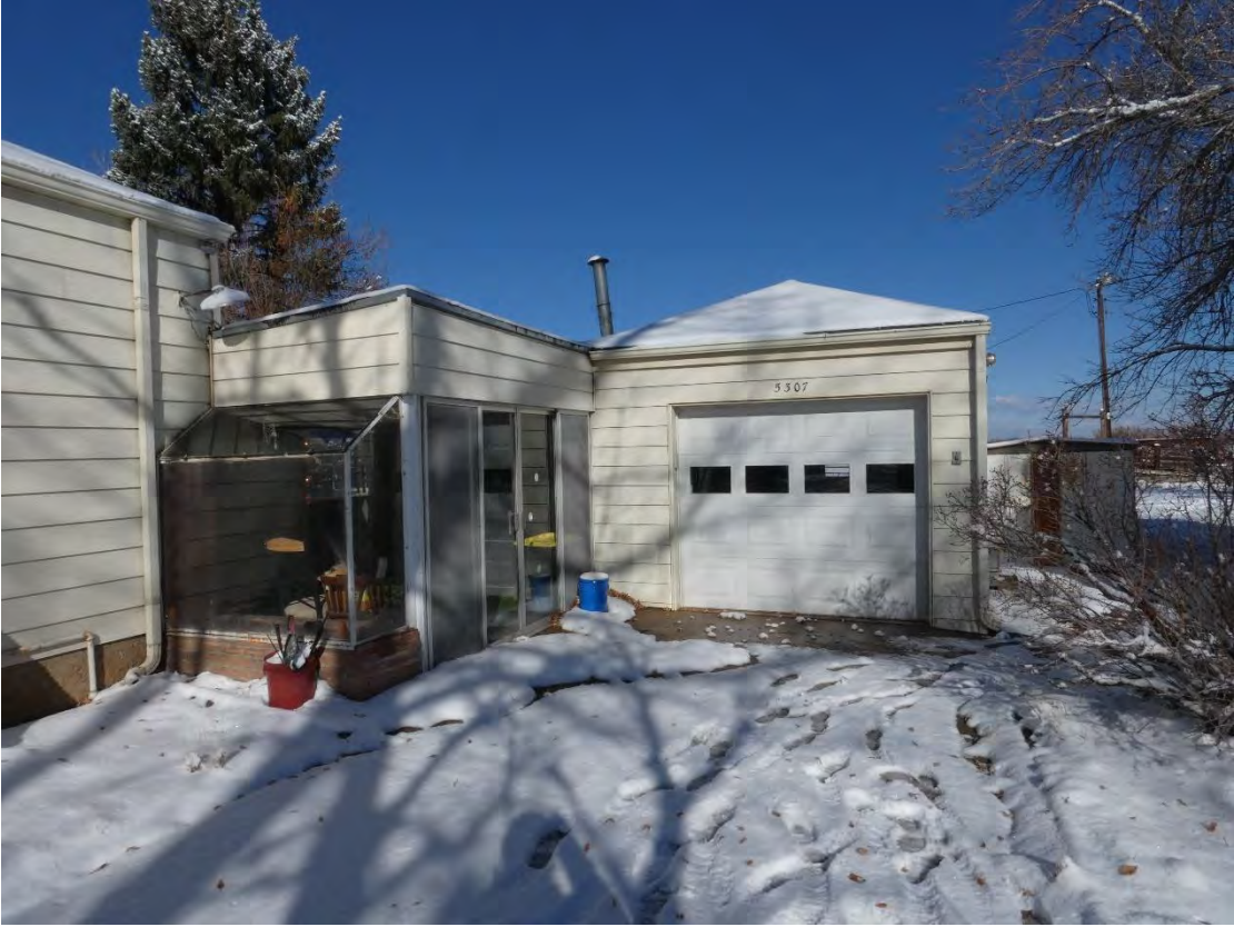
1950s Garage South Elevation
