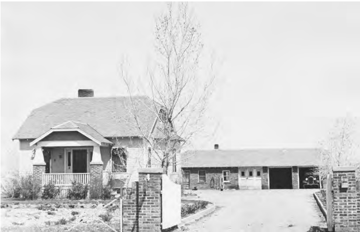
Original Residence and Garage South Elevation 5307 Independence Road 1930-1949 Carnegie Library for Local History BHS 207-28-38
