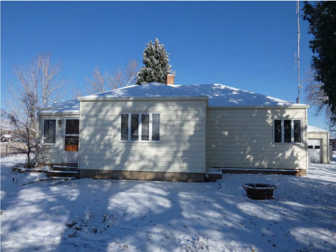
1950s Residence South Elevation
