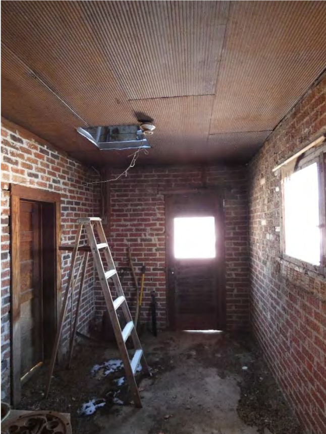
Original Garage Interior Back Room
