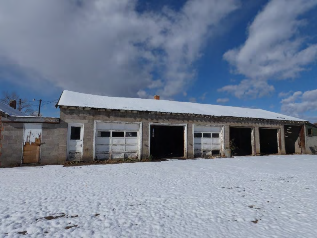
Original Garage Addition East Elevation
