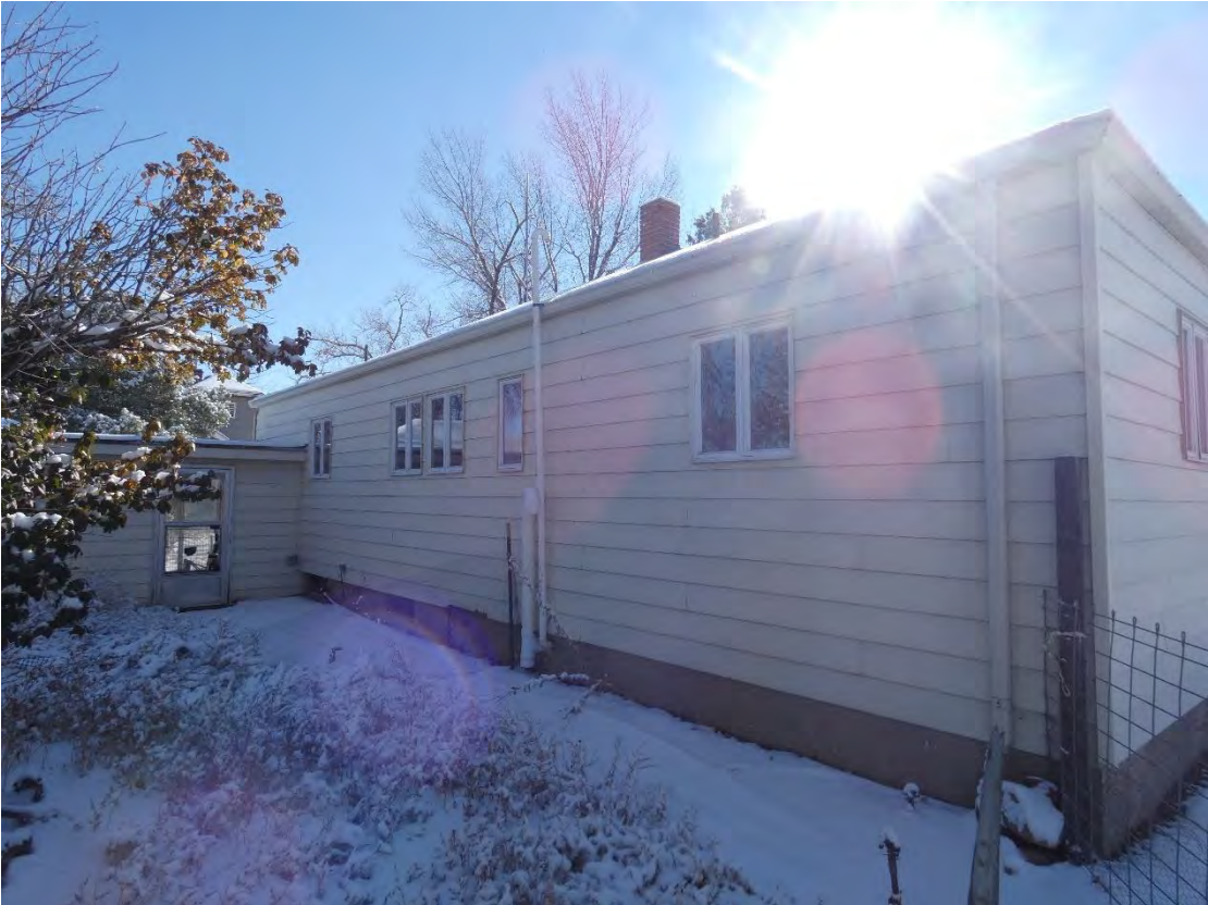
1950s Residence North Elevation
