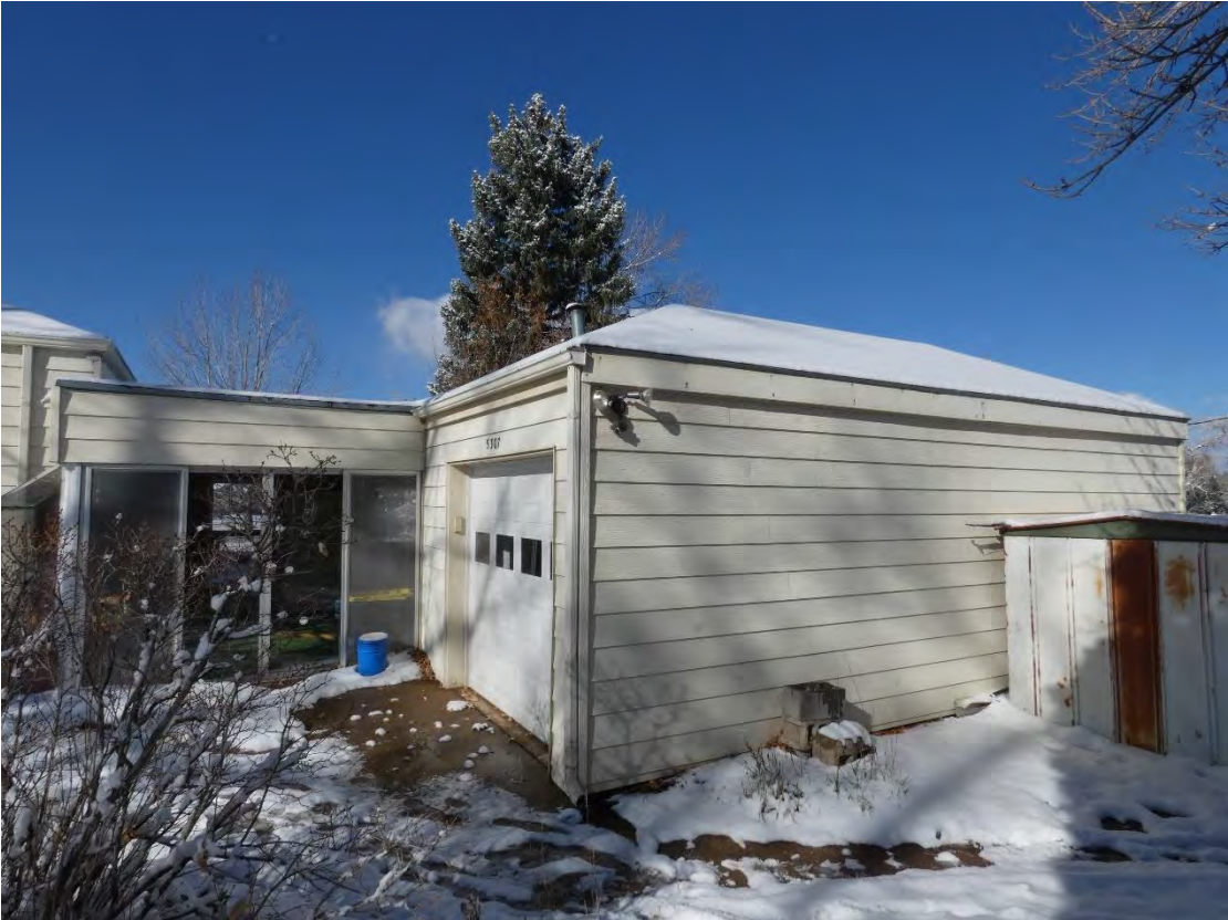
1950s Garage East Elevation
