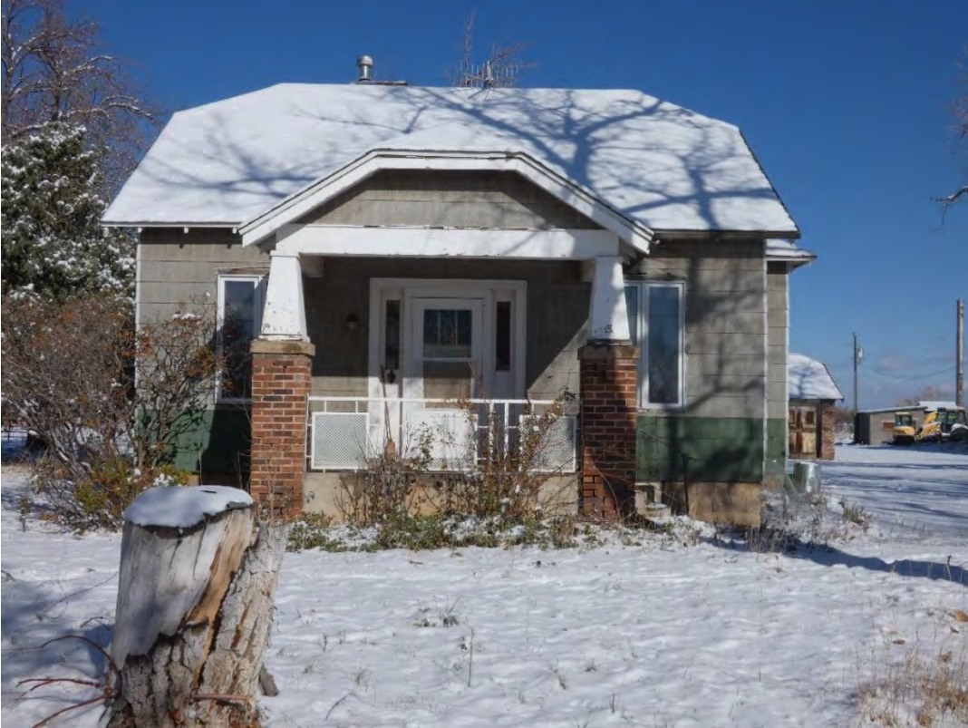
Original Residence South Elevation
