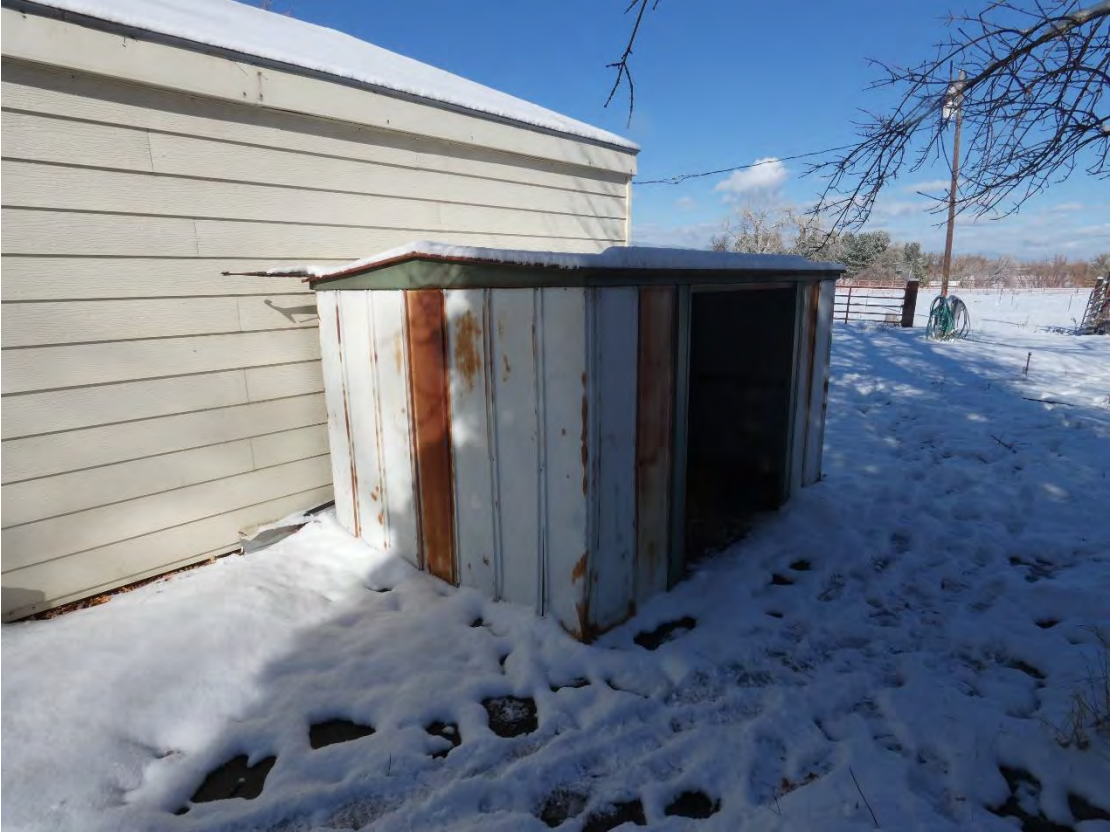
Metal Shed Southeast Elevation
