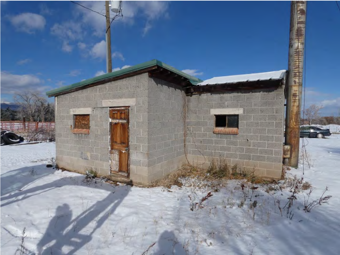
Concrete Shed South Elevation
