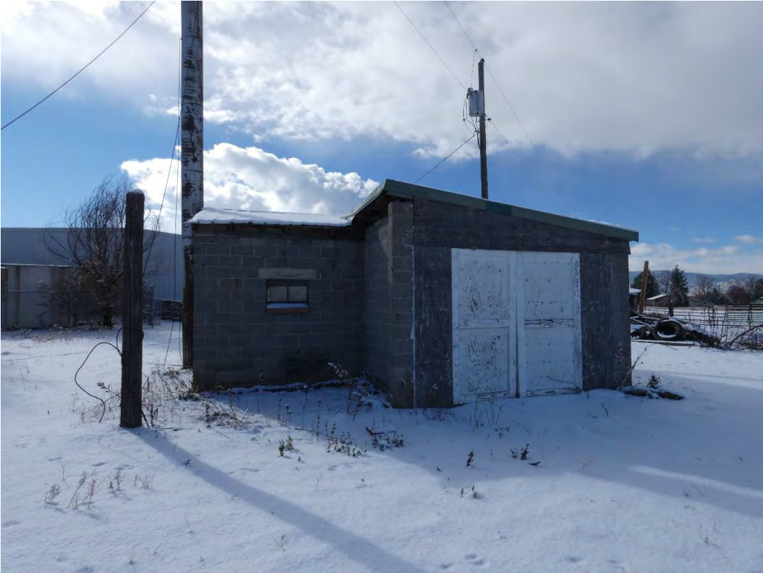
Concrete Shed North Elevation
