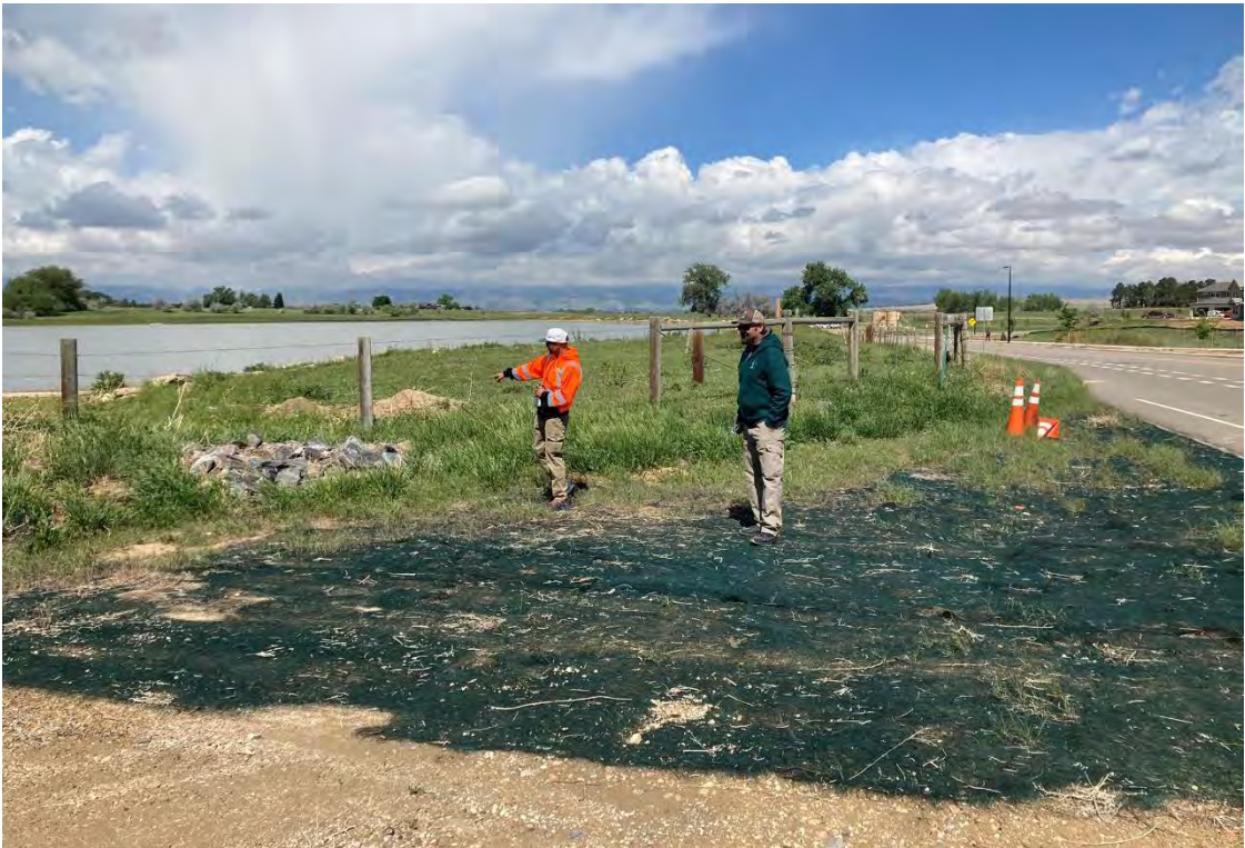
Staff pointing toward riprap at existing spillway. Spillway to be modernized and increased to 90-foot width. This area will also serve a one of the staging areas. N.111 th Street visible on right side of photo.
