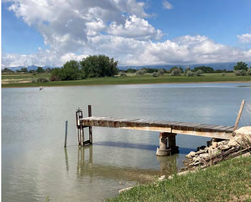
(Left) Bridge access to gate that opens outlet for discharging water from reservoir. New outlet works are planned for this location.
