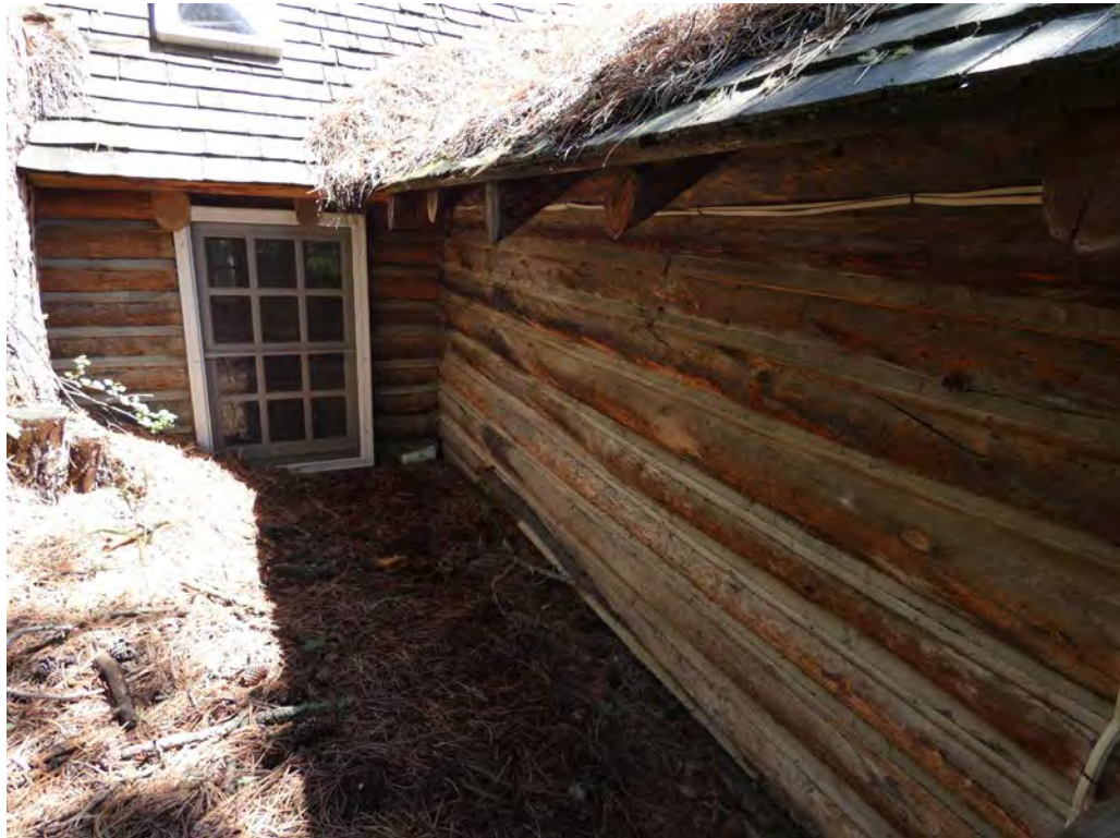
Cabin 3: northwest elevation
