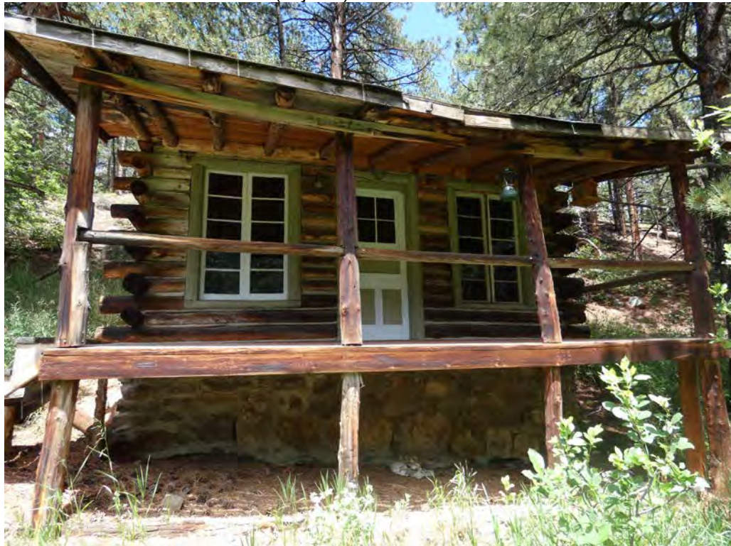
Cabin 3: southeast elevation (façade)
