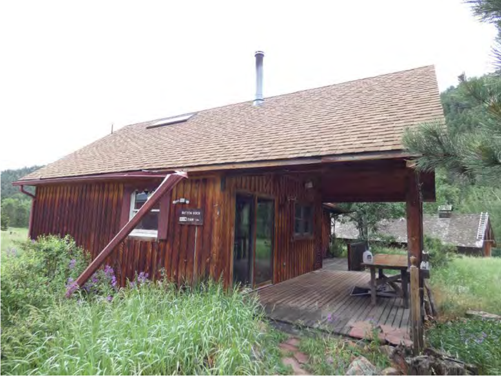
House: northeast elevation
