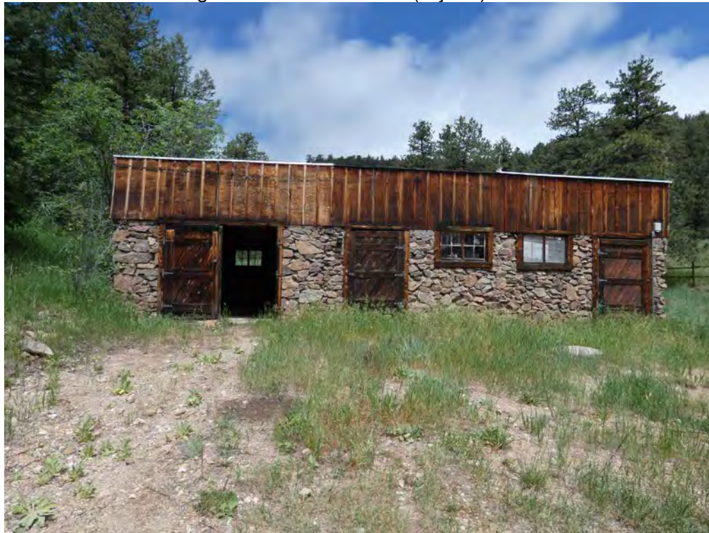
Stone Barn and Garage: southeast elevation (façade)
