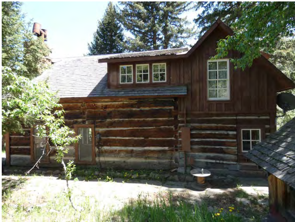
Cabin 1: northwest elevation
