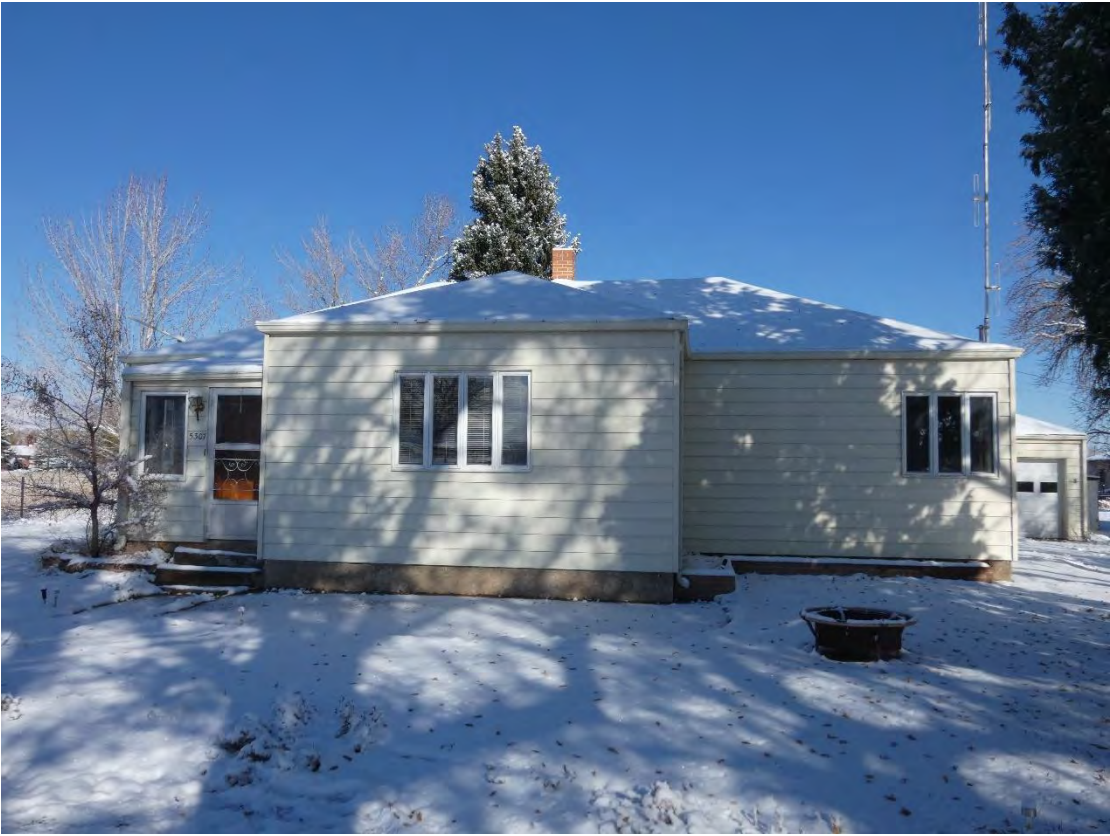
1950s Residence South Elevation
