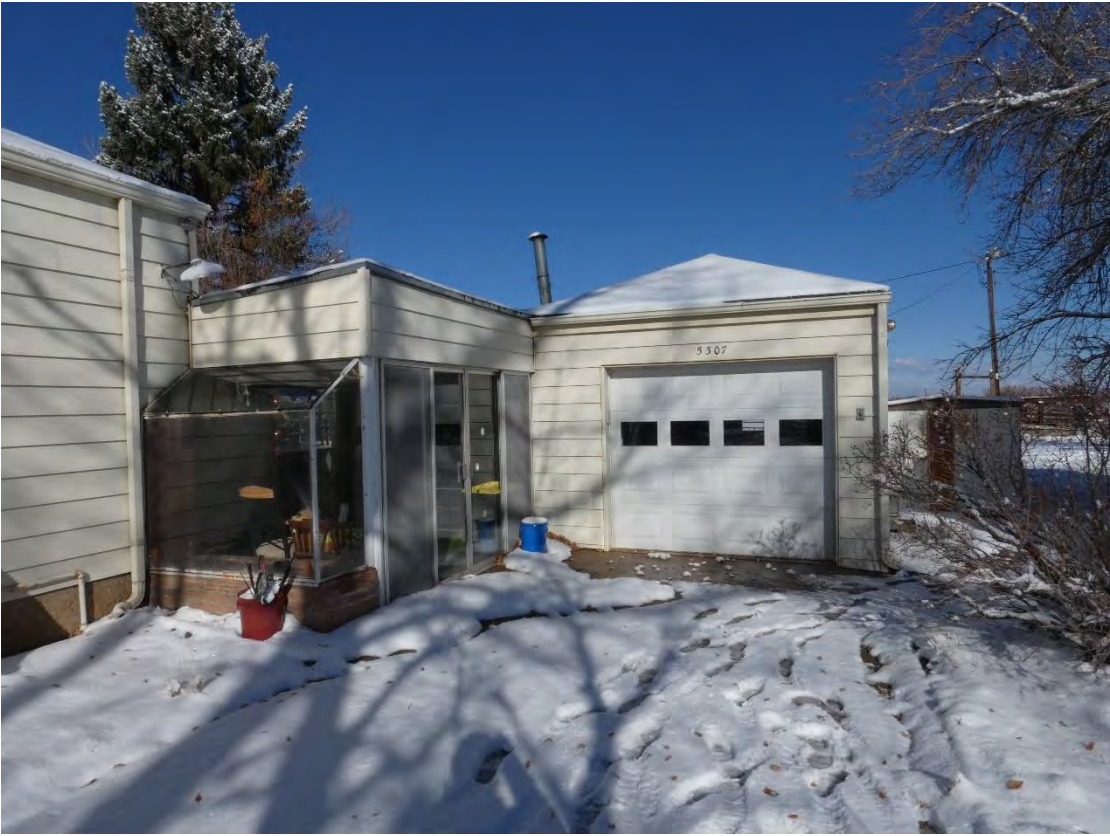
1950s Garage South Elevation
