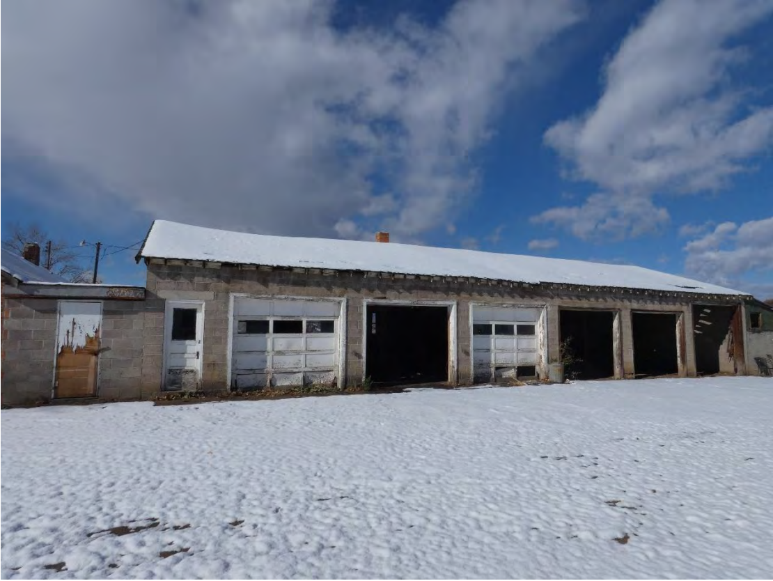
Original Garage Addition East Elevation
