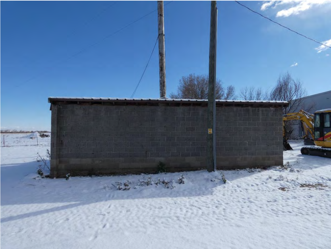
Concrete Shed West Elevation
