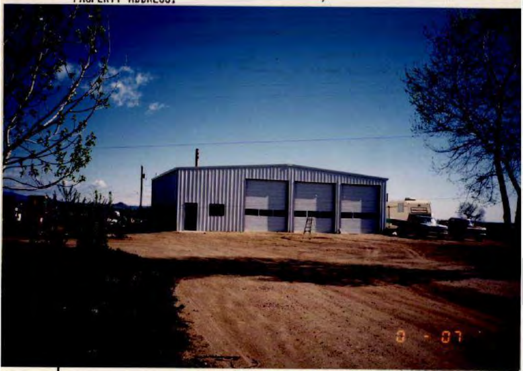
Large Garage South Elevation Assessor's Photo 1990
