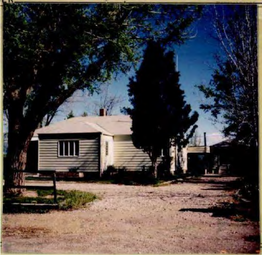
1950s Residence South Elevation Assessor's Photo Unknown Date
