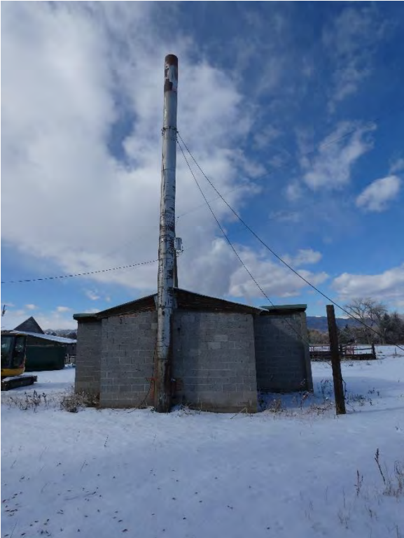
Concrete Shed East Elevation
