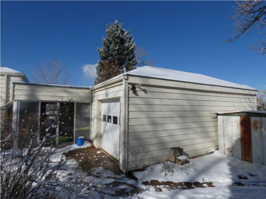
1950s Garage East Elevation
