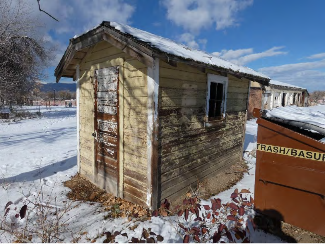
Wood Shed Southeast Elevation
