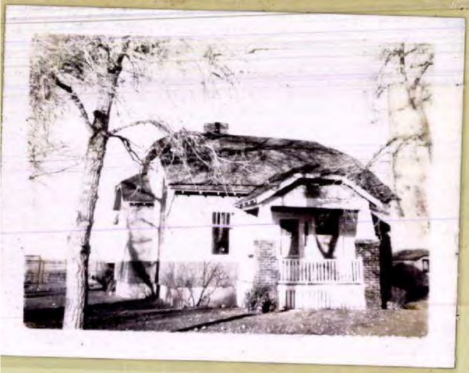
Original Residence South Elevation Assessor's Photo 1966
