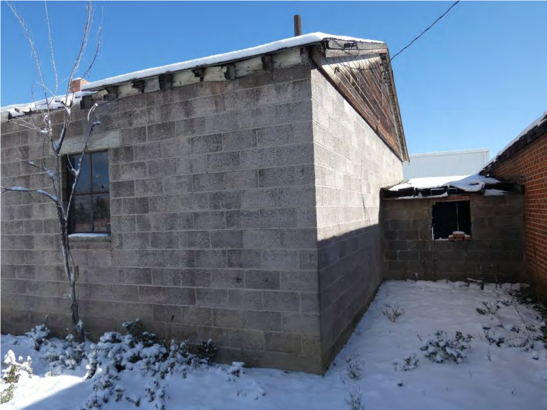
Original Garage Addition Southwest Elevation
