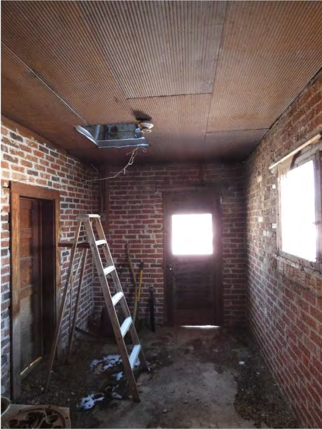
Original Garage Interior Back Room
