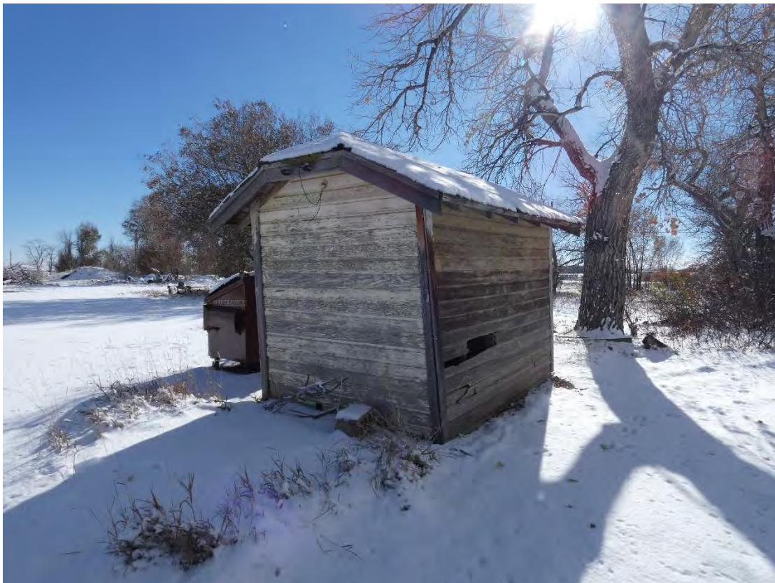
Wood Shed Northwest Elevation
