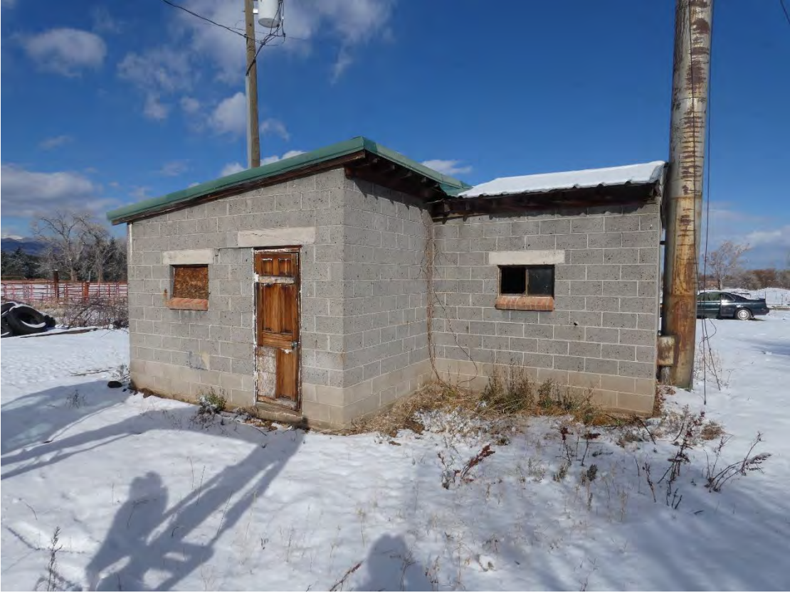
Concrete Shed South Elevation
