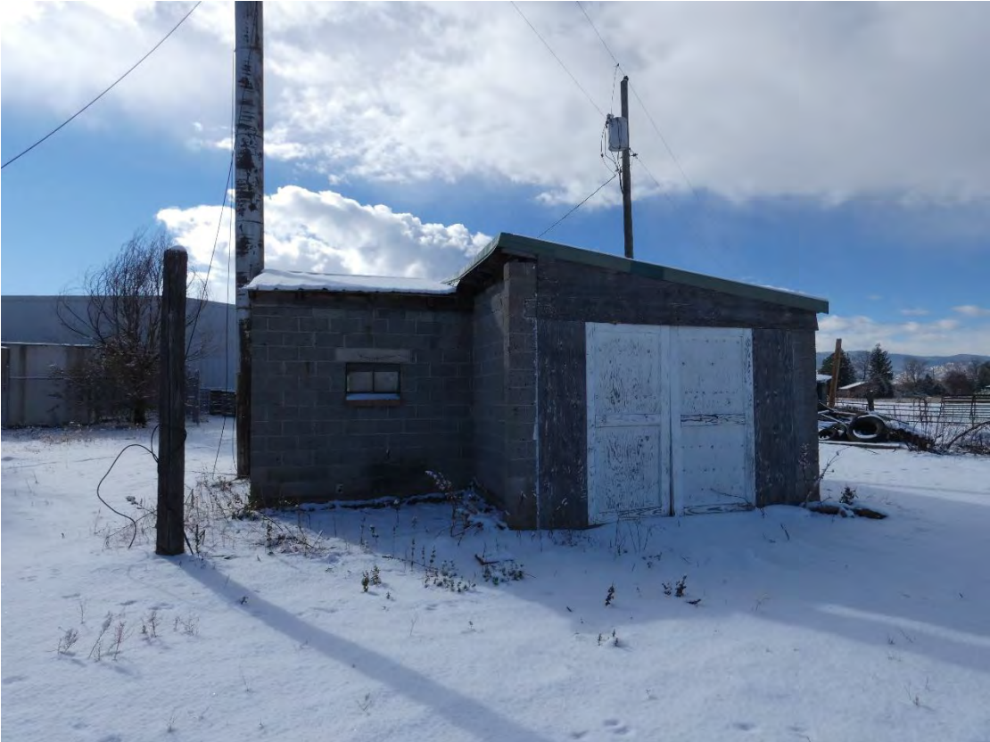
Concrete Shed North Elevation
