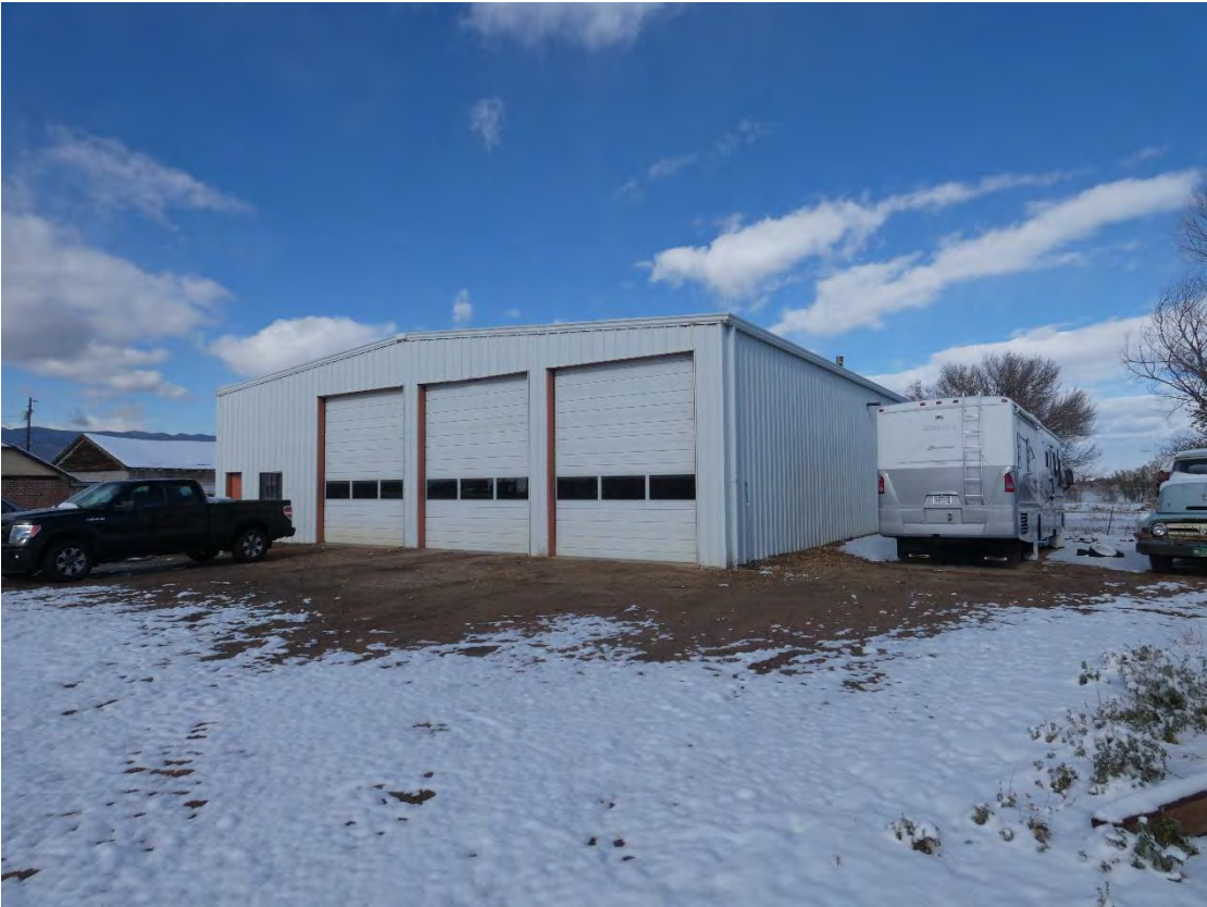
Large Garage Southeast Elevation
