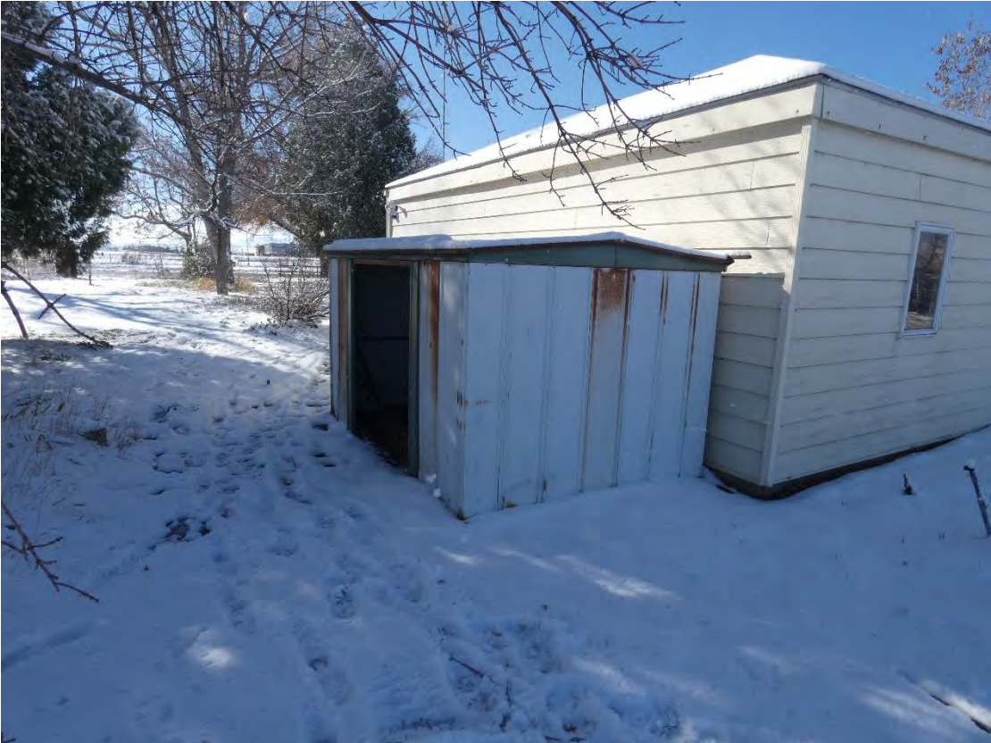
Metal Shed Northeast Elevation
