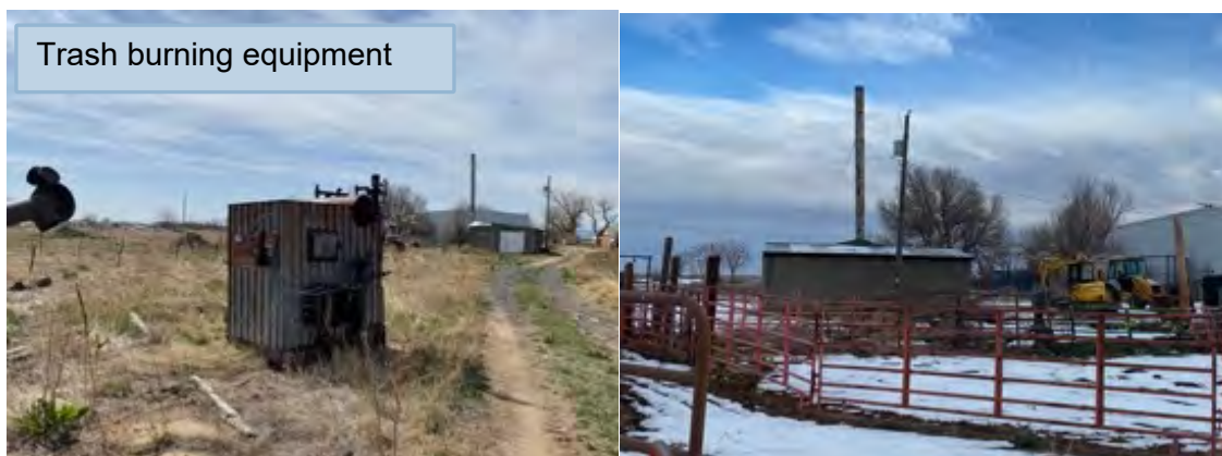
Boiler, smokestack and buildings are to be removed
