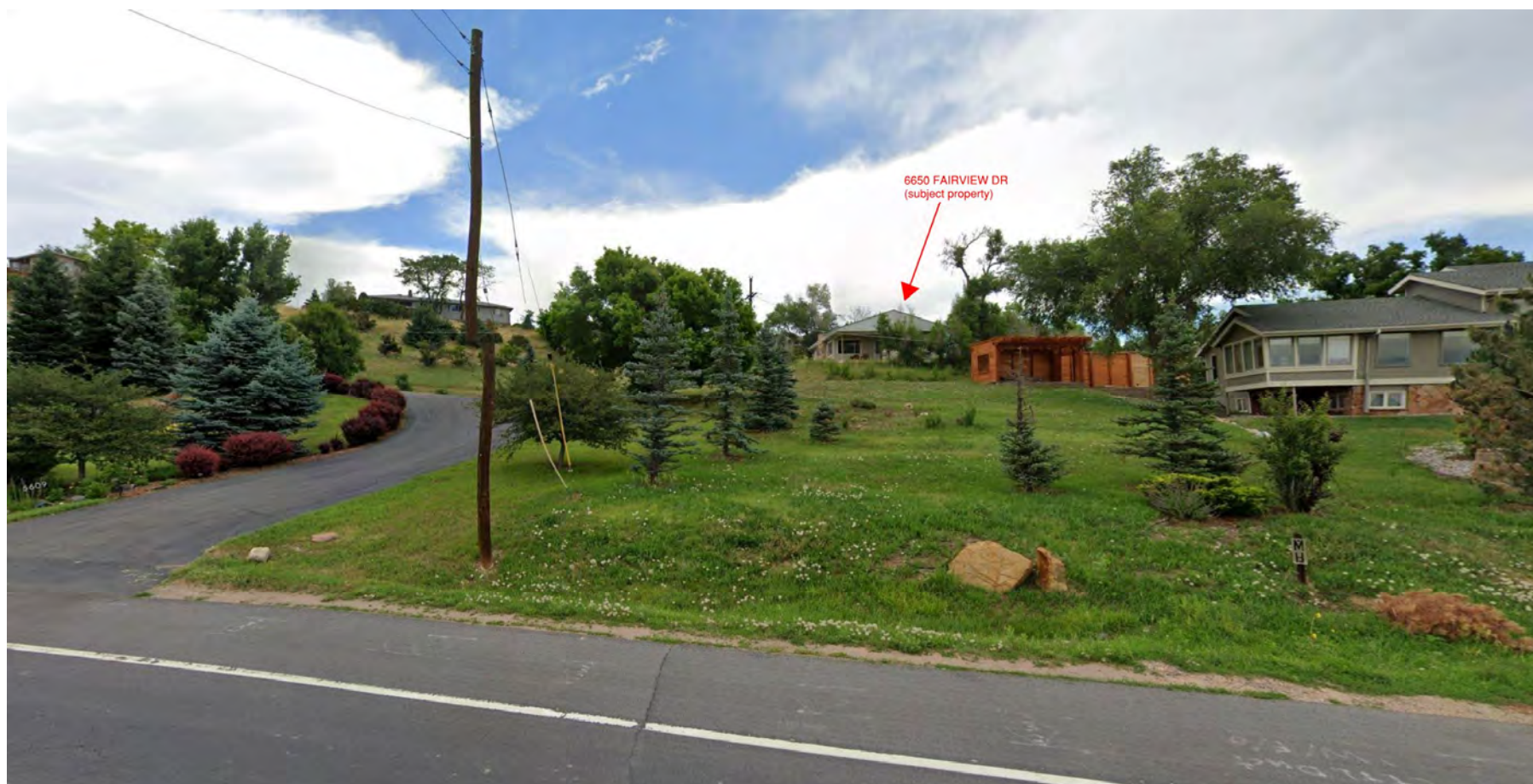
4. View of existing house at 6650 Fairview Drive from Baseline Road looking North
