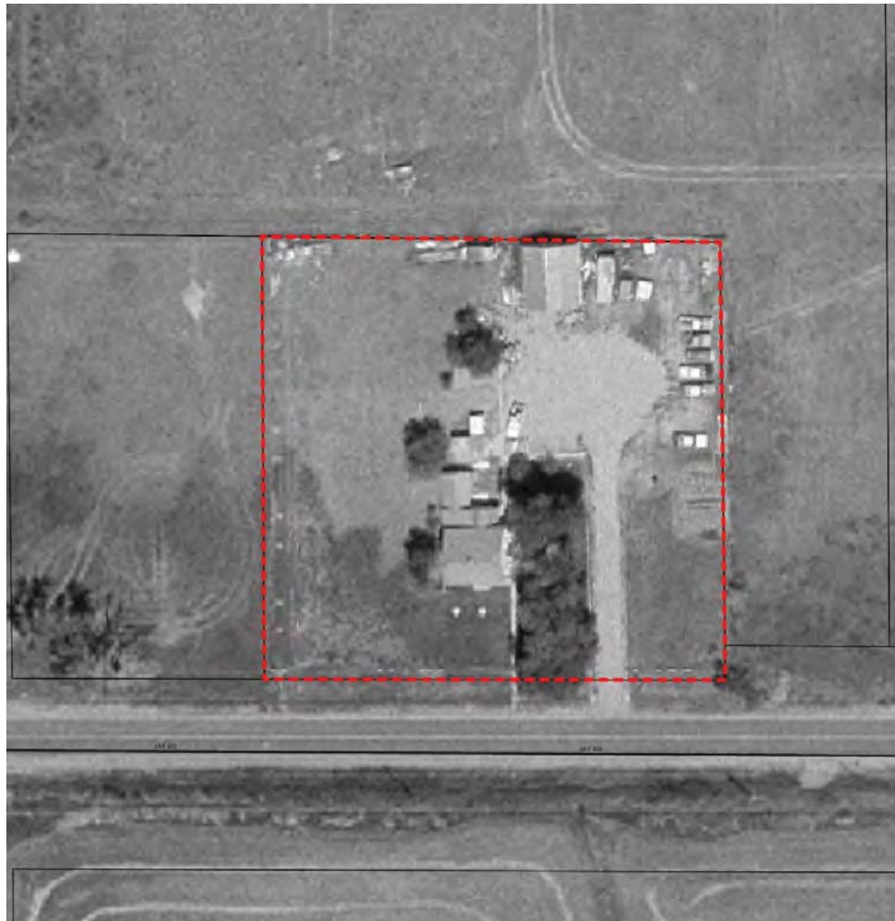
Figure 1: 1977 Aerial photo of subject parcel, no covered porch shown on the south side of the residence.
