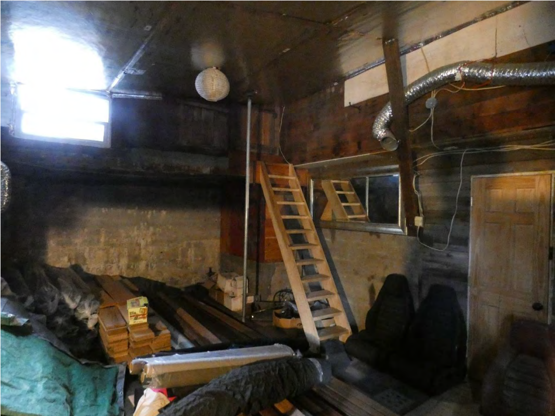
Interior- Center Room Garage and 2nd Story Apartment February 2023
