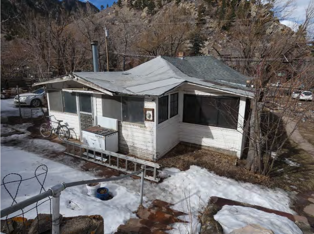
House South Elevation February 2023
