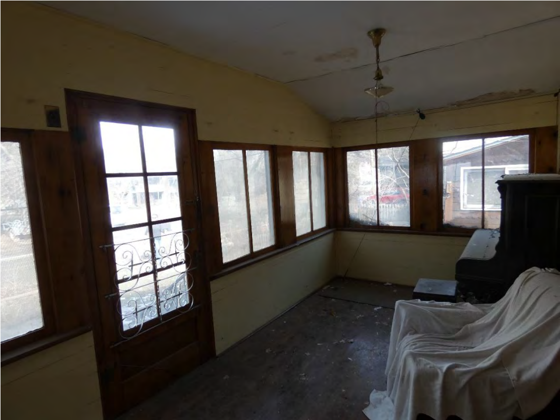
House Interior -North Closed in Porch February 2023
