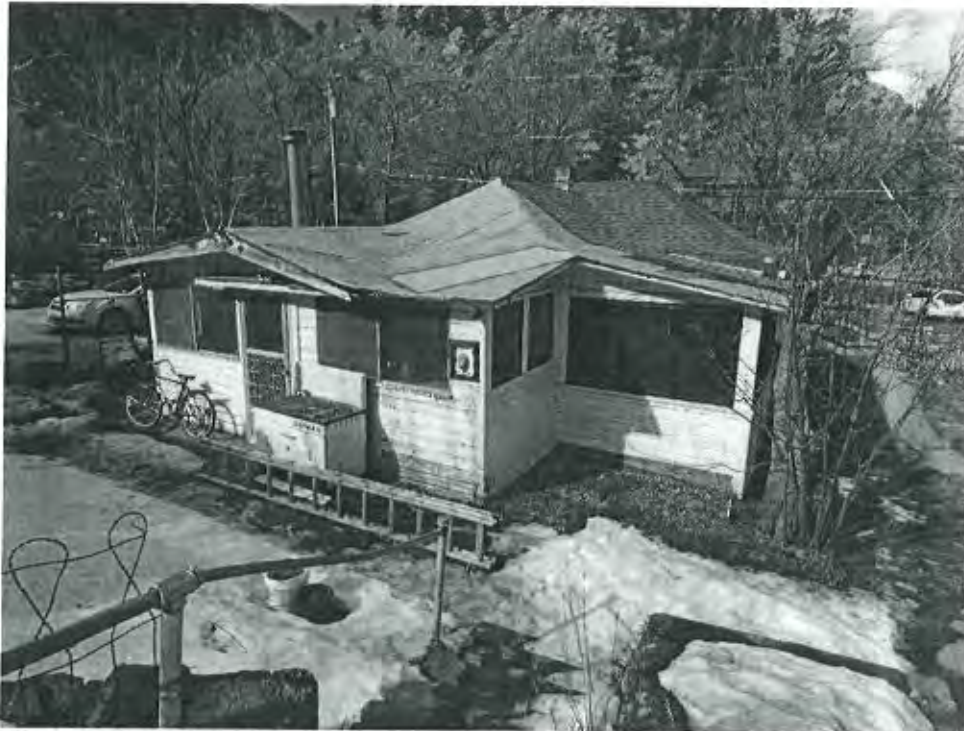
House South Elevation February 2023
