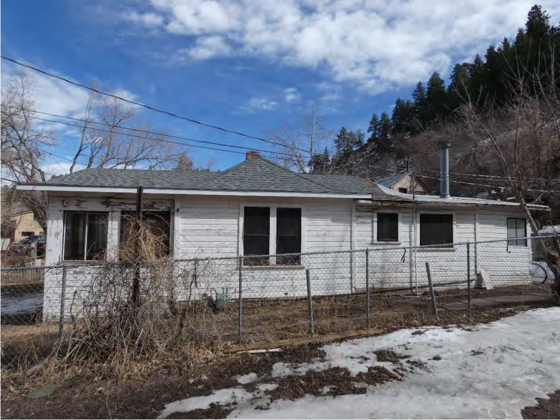
House West Elevation February 2023
