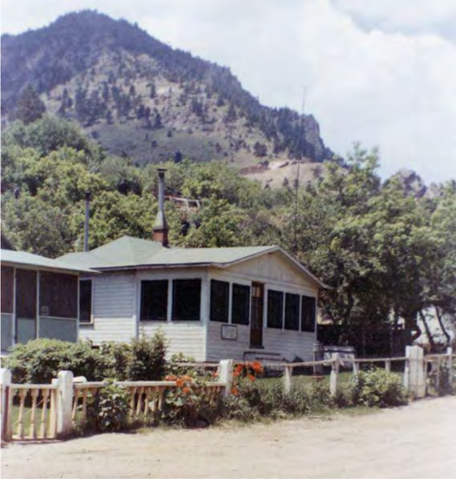
House Northeast Elevation Photo 4. A Kodacolor photograph looking south and west at the Chesebro home. Dated August 1961. Note the weather gauge is in the front lawn near the fence. Eldorado Springs: Chesebro properties Carnegie Library Call Number 701-2-16
