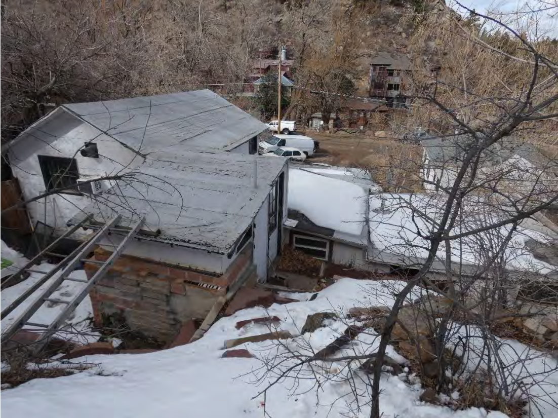
Garage and 2nd Story Apartment South Elevation February 2023
