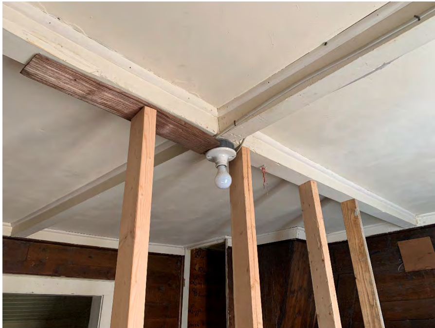
Figure 102: Light fixture located in the center of the living room ceiling.
