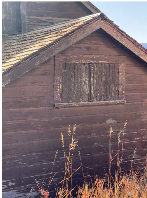
Figure 33: Typical exterior wood siding and trim.
