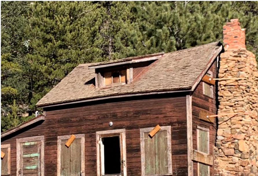
Figure 42: Overall view of the west side of the cabin roof.
