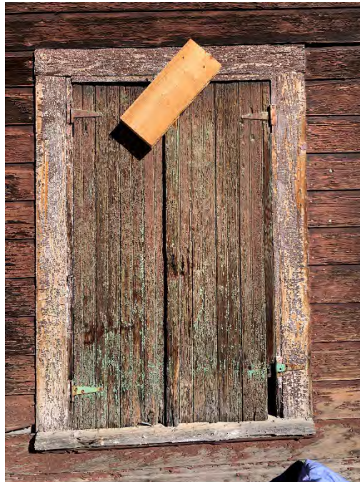
Figure 58: Exterior view of typical shutters.
