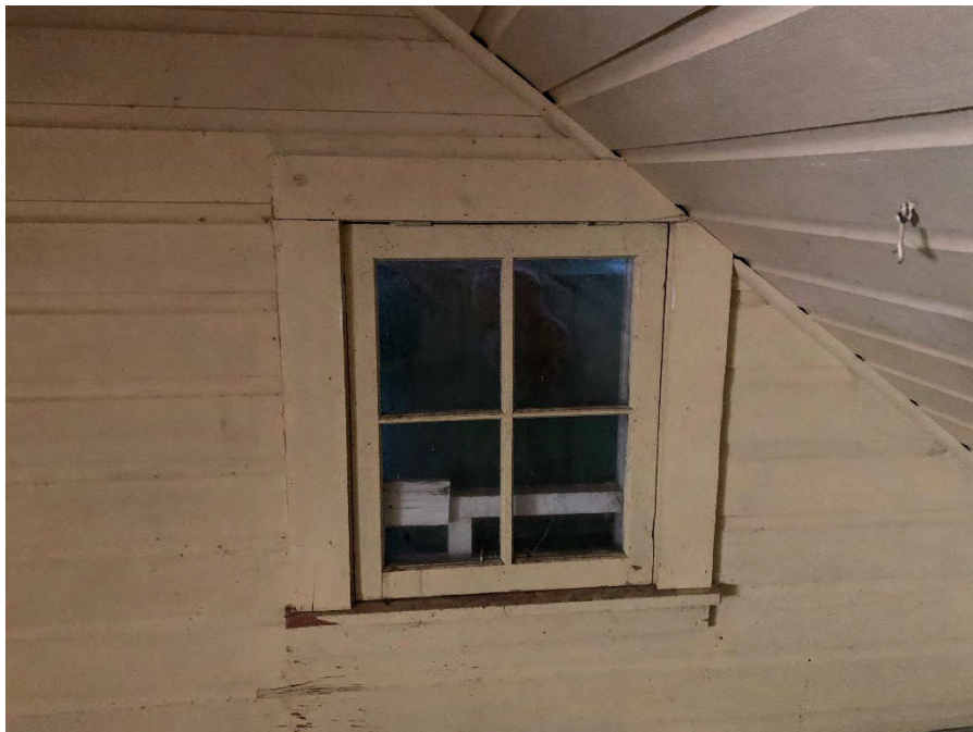
Figure 71: Interior view of typical south elevation second floor windows.
