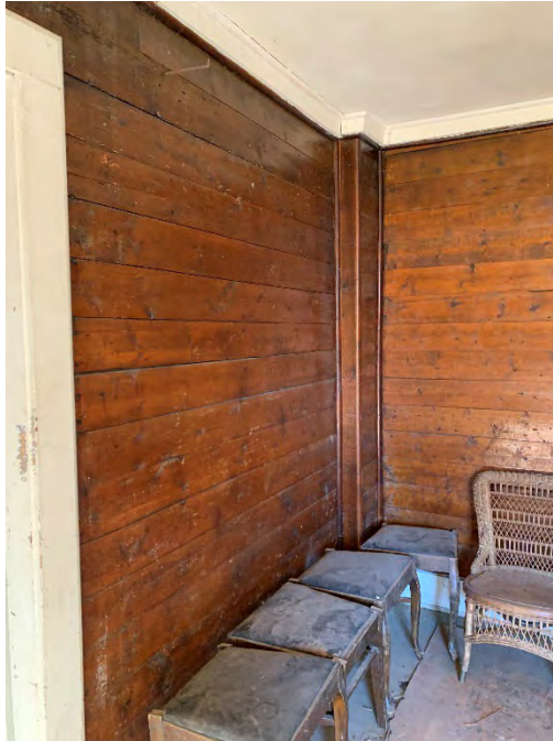
Figure 72: Horizontal wood plank wall finish in the first floor living room.
