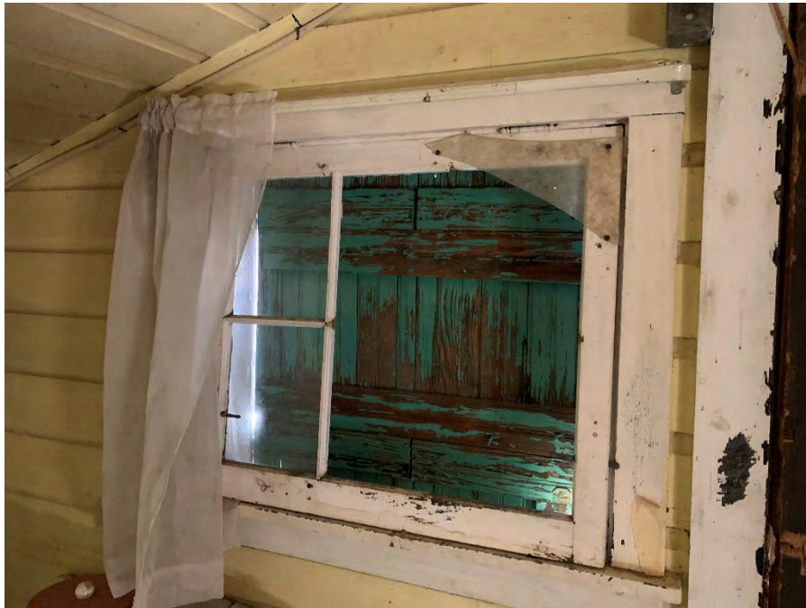
Figure 68: Interior view of Window 109.
