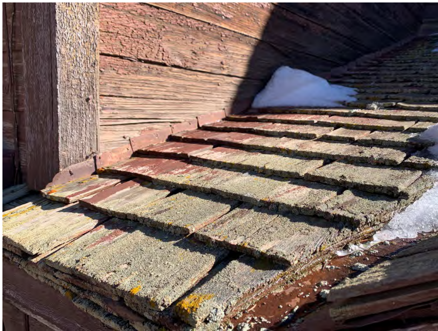
Figure 47: Detail view of flashing at roof to wall transition.
