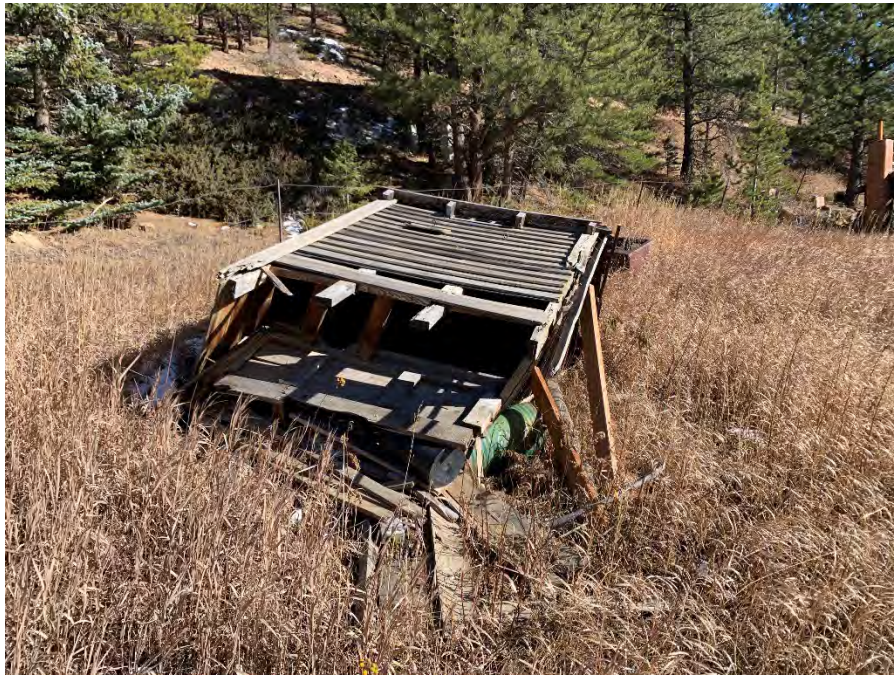
Figure 15: Outhouse located to the north of the cabin.
