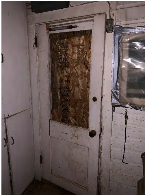
Figure 54: Interior view of north elevation door.
