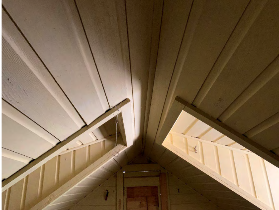
Figure 82: Ceiling finish typical in the second floor bedroom.
