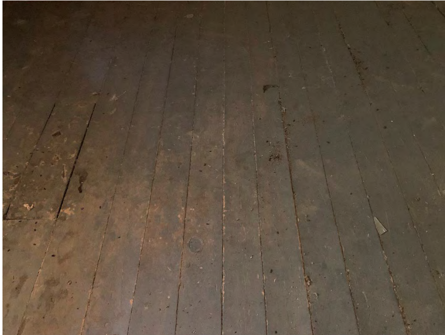
Figure 85: Wood plank flooring in the second floor bedroom.
