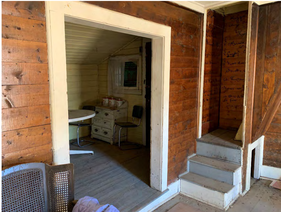
Figure 94: Painted wood casing, trim, and stairs located in the living room.
