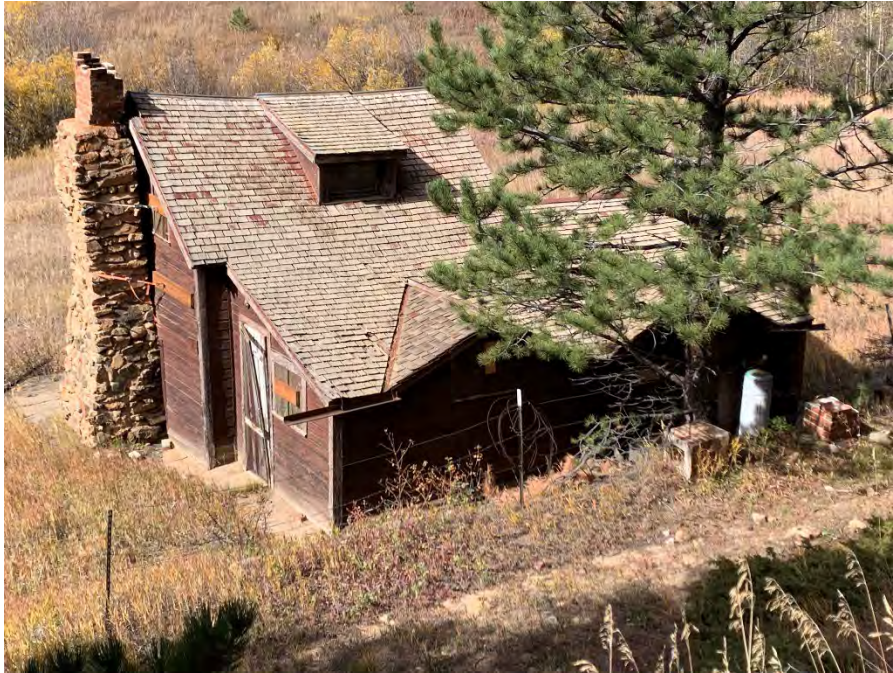
Figure 41: Overall view of the east side of the cabin roof.
