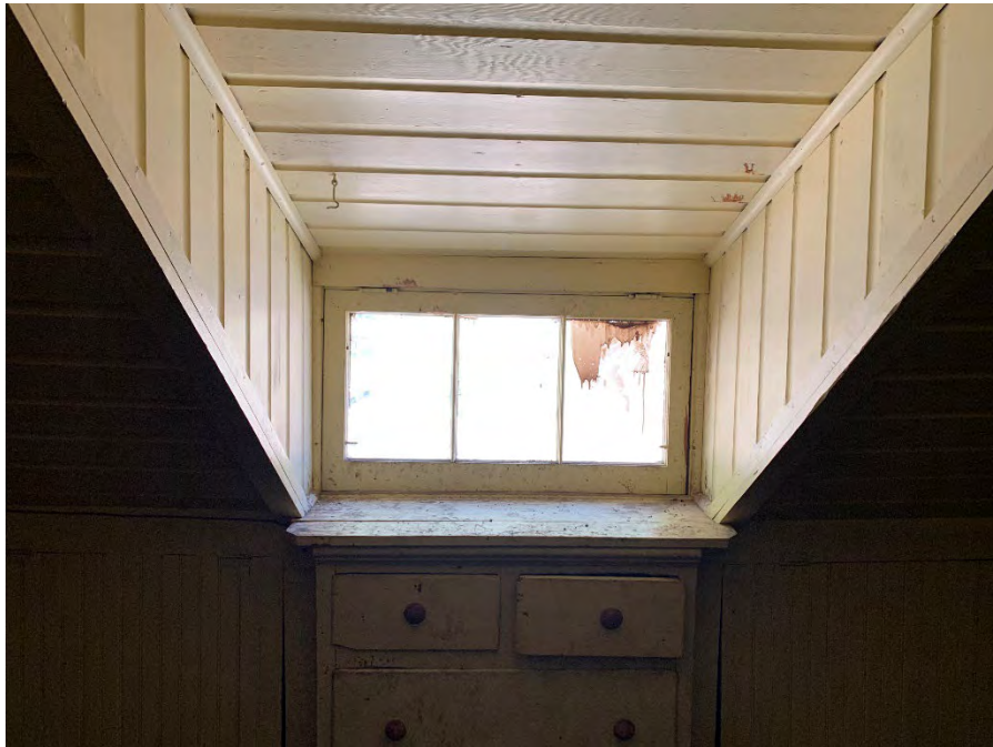
Figure 70: Interior view of second floor dormer window.
