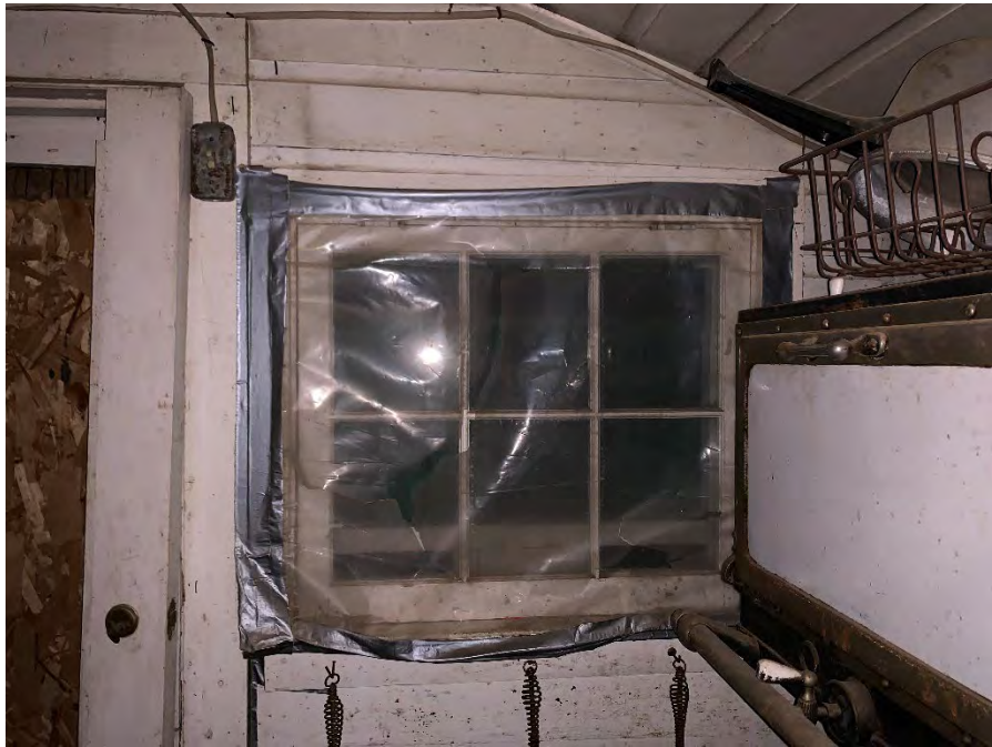
Figure 64: Interior view of Window 105.
