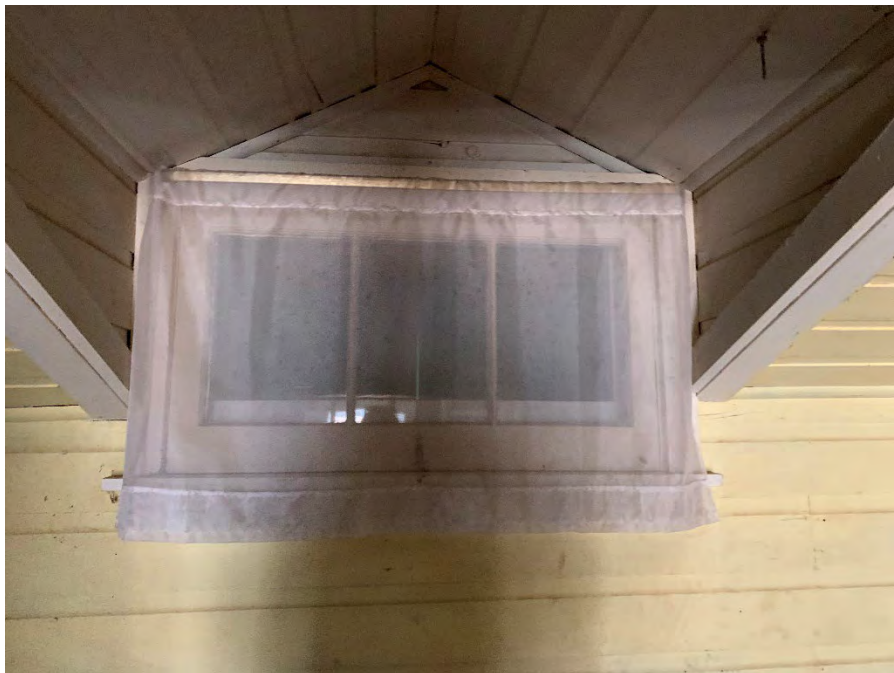
Figure 67: Interior view of Window 108.
