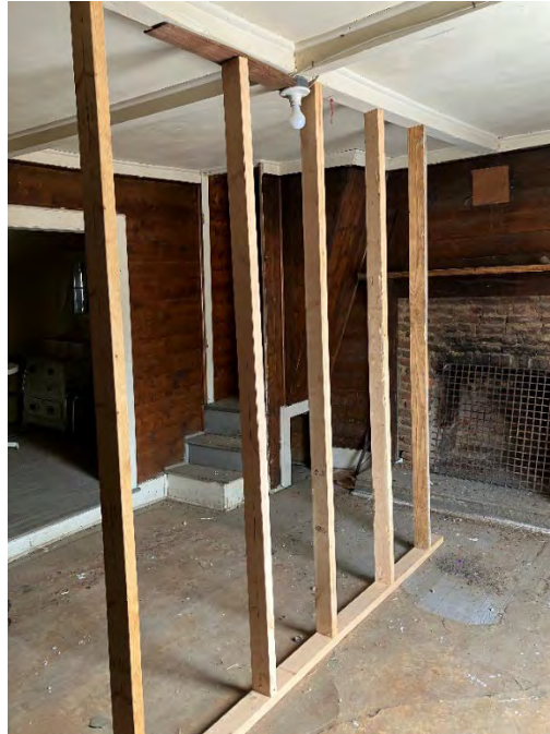
Figure 27: Temporary stud shoring wall supporting second floor framing above
