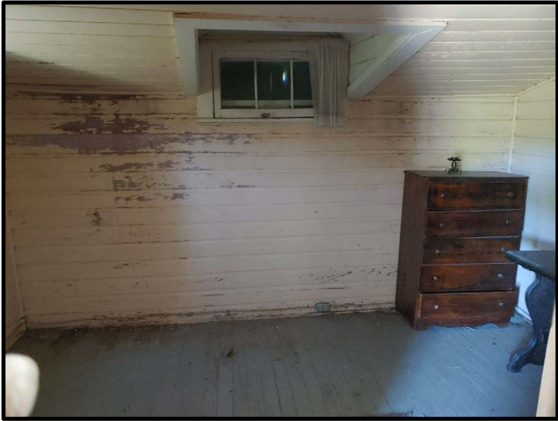
Tucker Cabin – 1 st floor bedroom after interior cleanup
