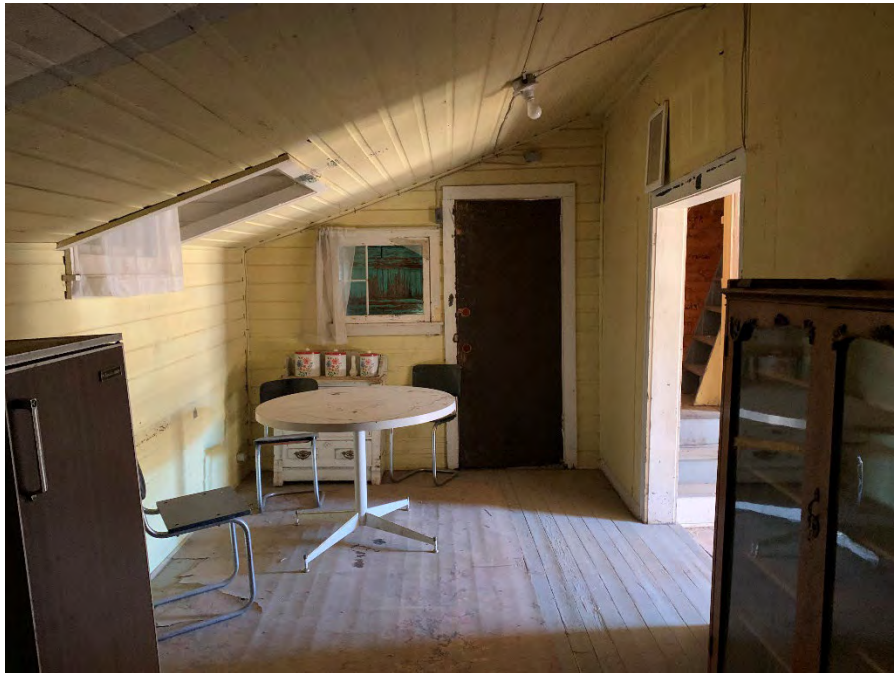
Figure 75: Overall view of the kitchen facing south.
