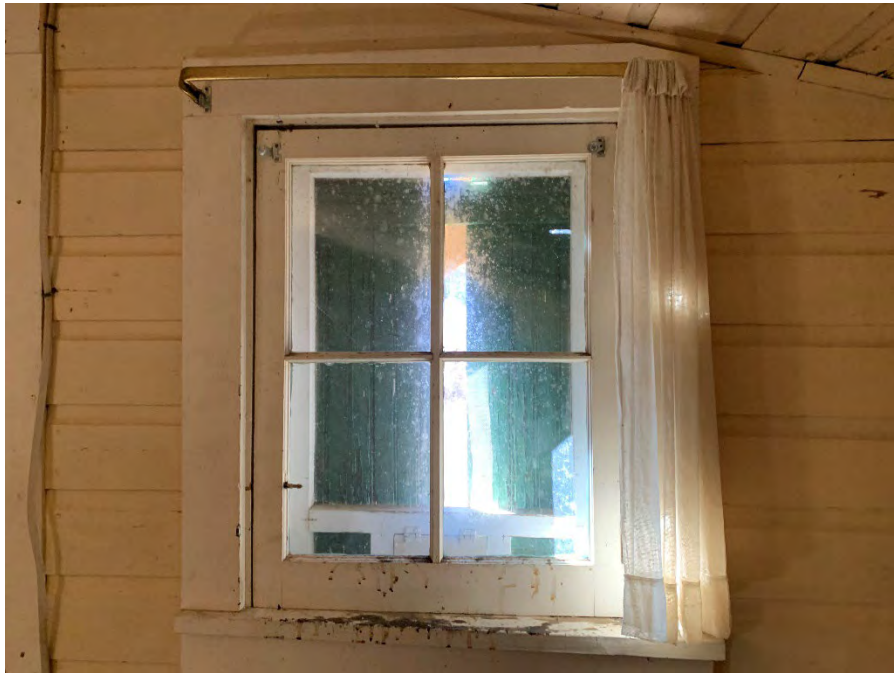
Figure 62: Interior view of Window 103.
