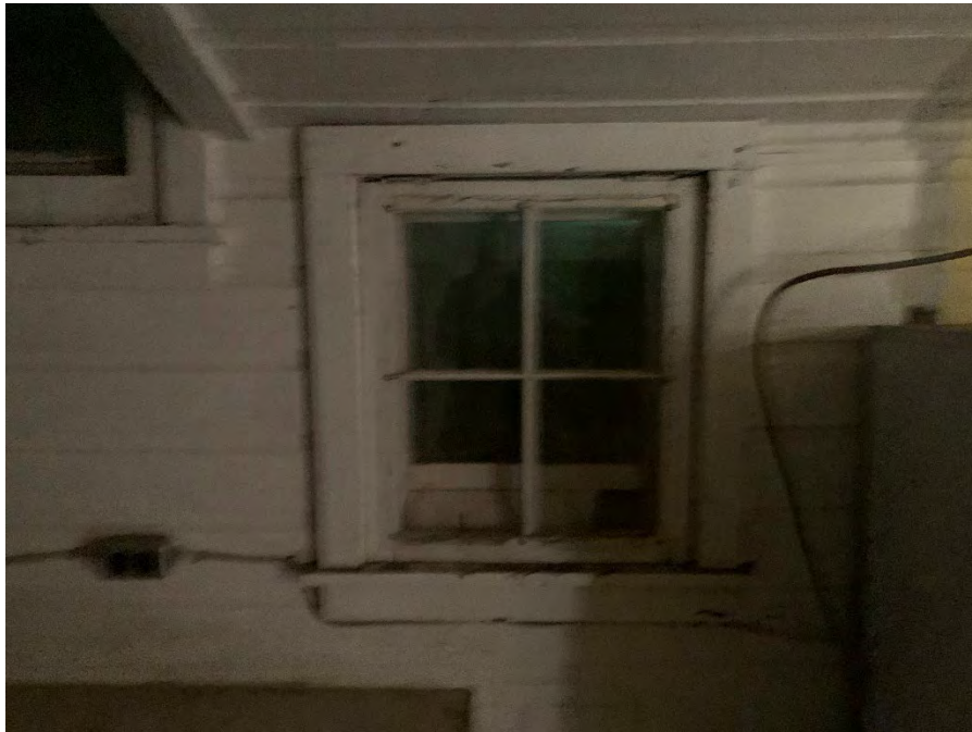
Figure 66: Interior view of Window 107.
