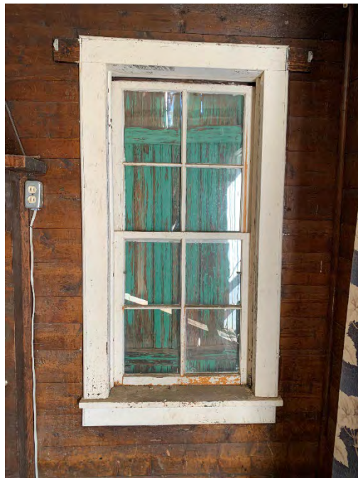
Figure 69: Interior view of Window 110.
