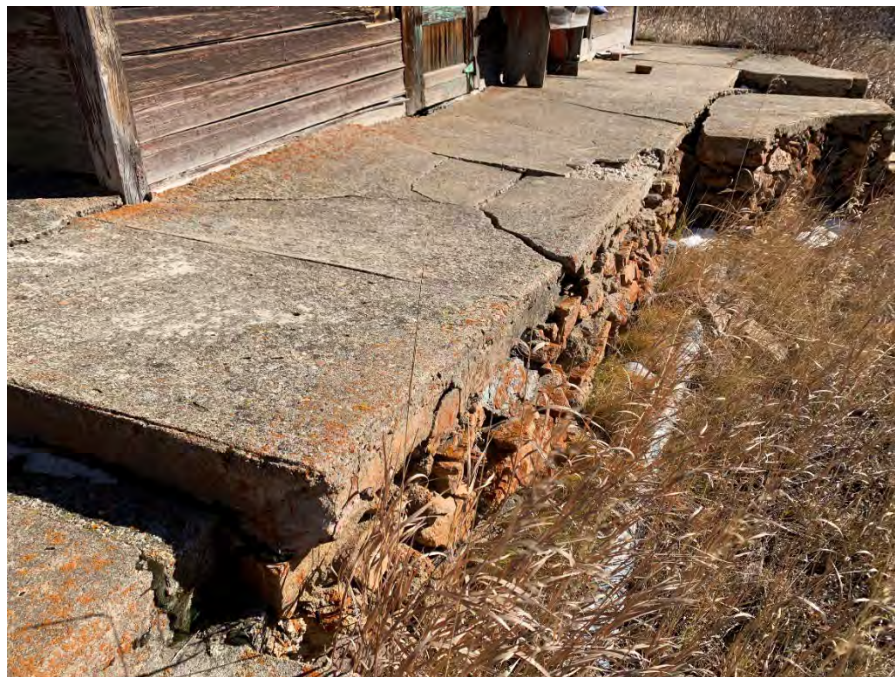
Figure 25: Rubble masonry platform and concrete topping at west elevation
