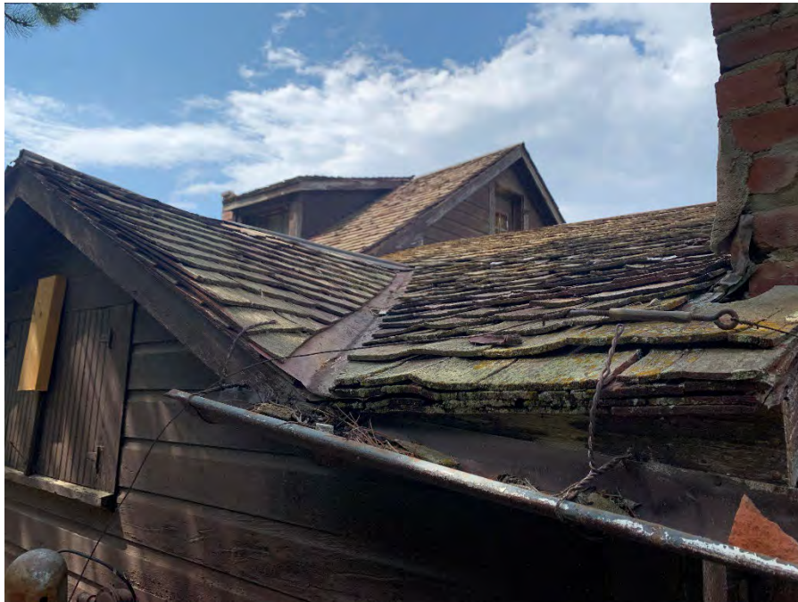
Figure 48: Half round gutter at the north end of the east elevation.
