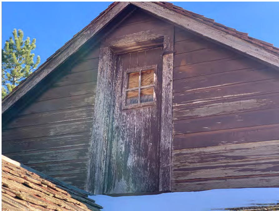
Figure 57: Exterior view of second floor door.
