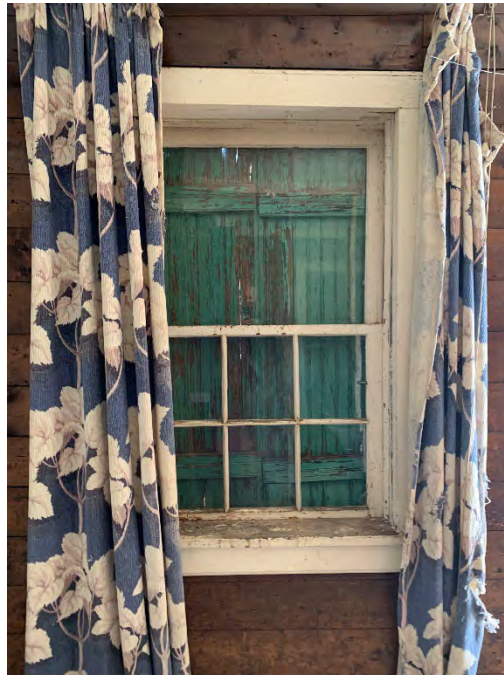
Figure 60: Interior view of Window 101.
