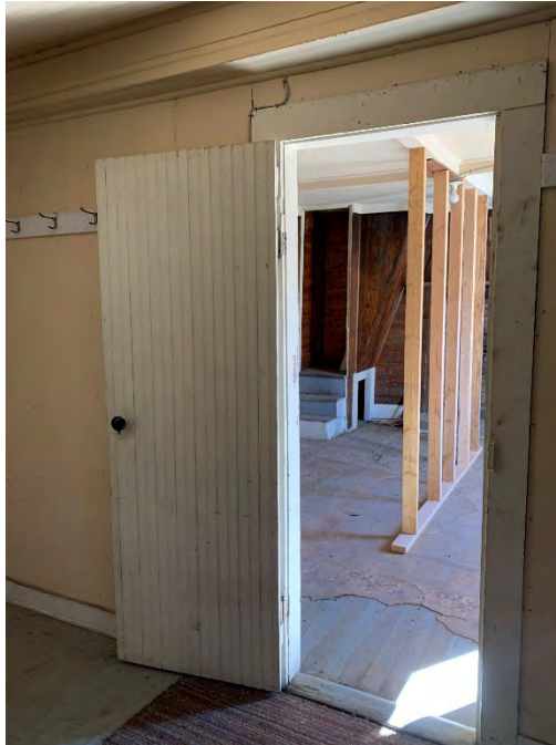
Figure 88: Door located between the first floor bedroom and the living room.
