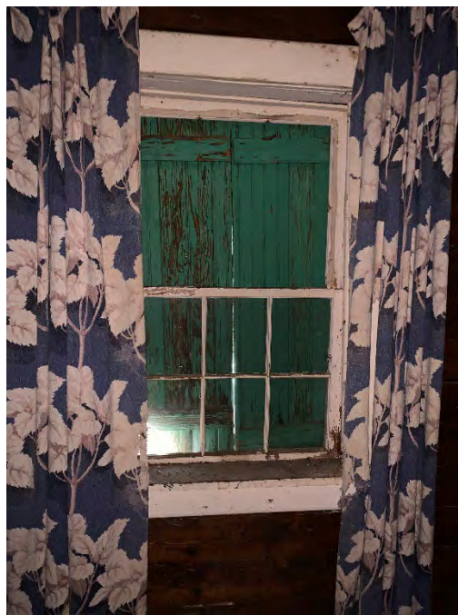
Figure 61: Interior view of Window 102.
