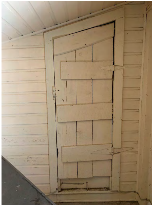
Figure 90: Door located between the first floor bedroom and the kitchen.
