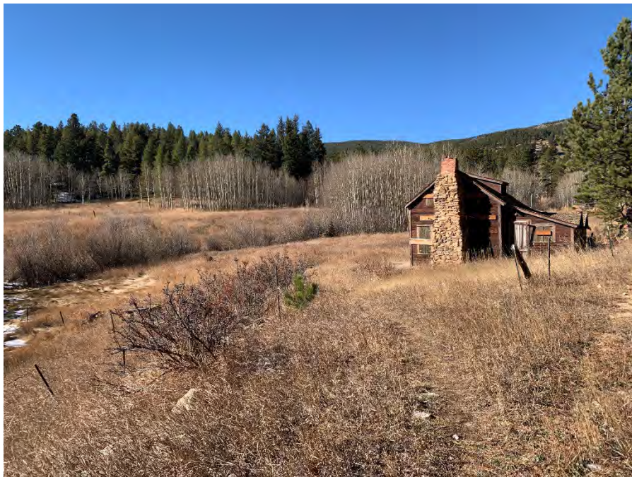
Figure 7: Overall view of the site from the south.
