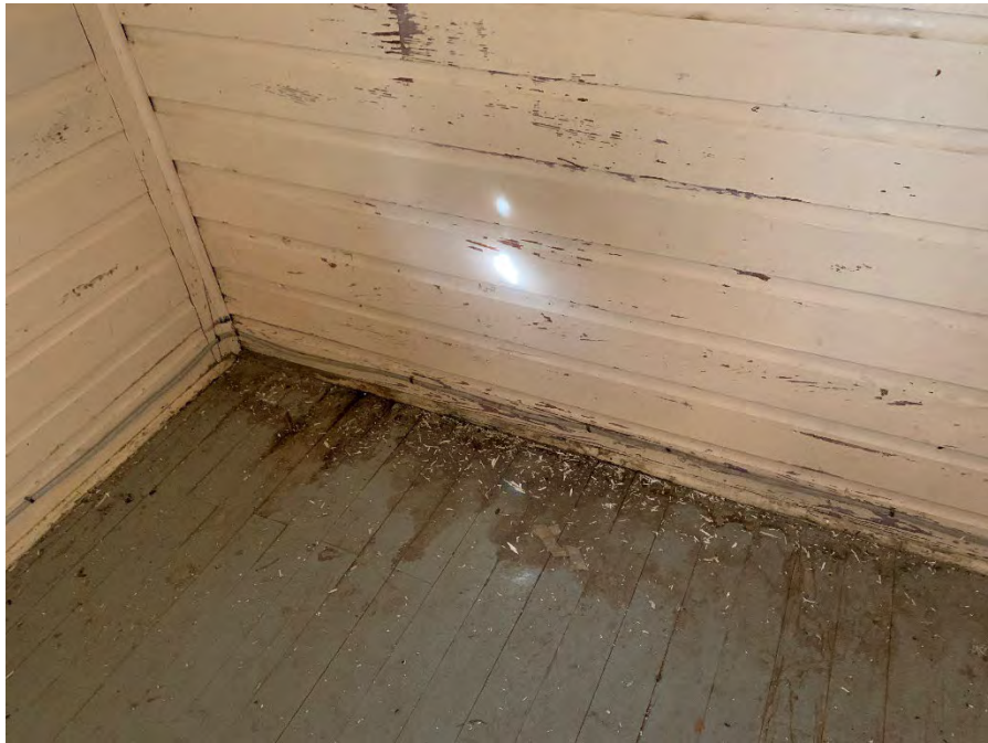
Figure 76: Wall and floor finishes in the first floor bedroom.
