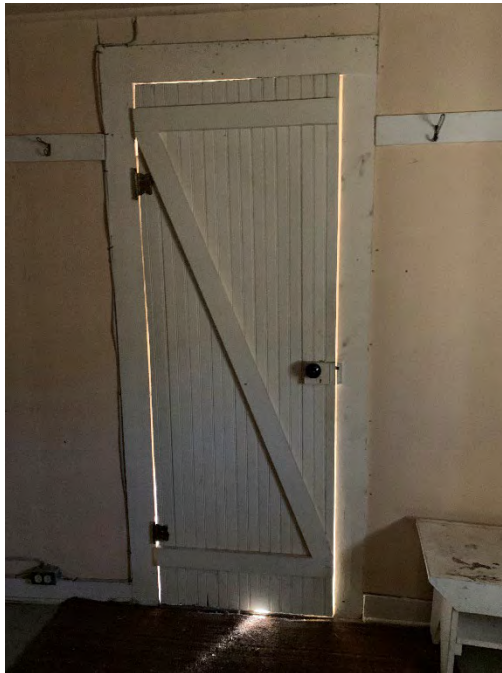
Figure 89: Door located between the first floor bedroom and living room.
