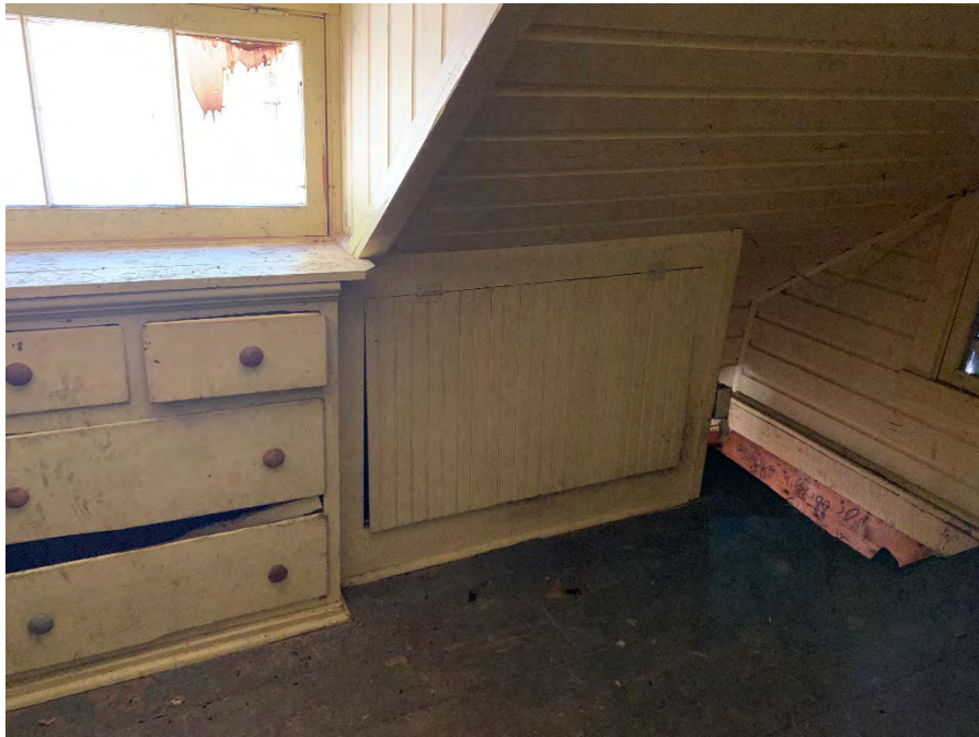
Figure 97: Storage area located in the second floor bedroom.
