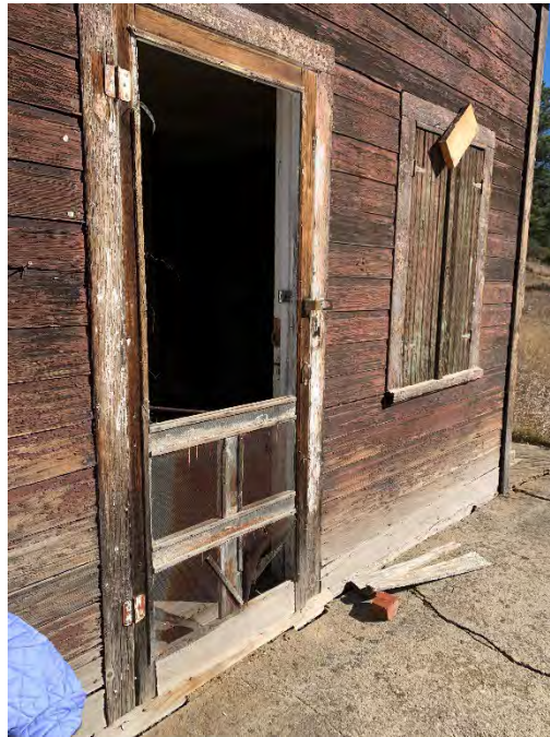
Figure 50: Exterior screen door at the main entrance on the west elevation.
