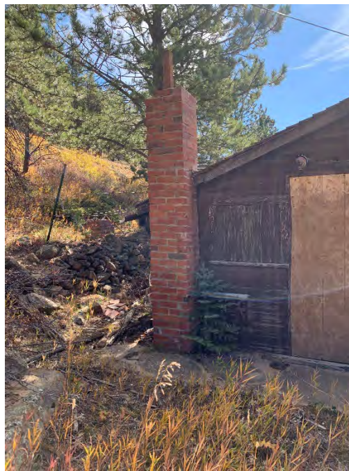
Figure 18: Site slope to the east of the building.
