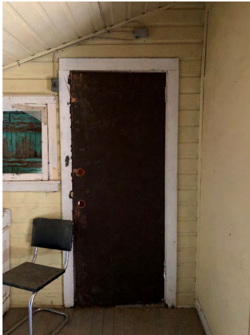
Figure 55: Interior view of south elevation door.
