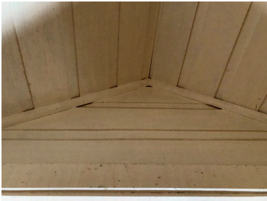
Figure 81: Ceiling finish in the first floor bedroom dormer.
