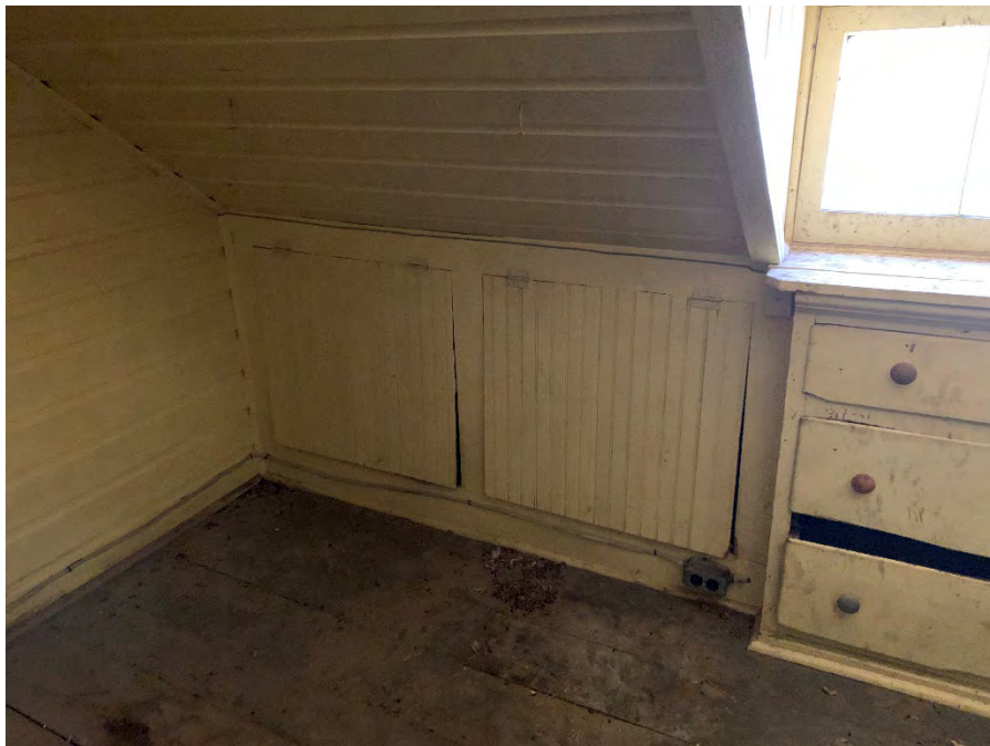
Figure 95: Second floor storage area.
