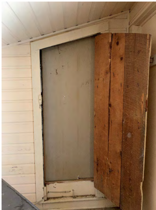
Figure 91: Door opening between the first floor bedroom and the kitchen.
