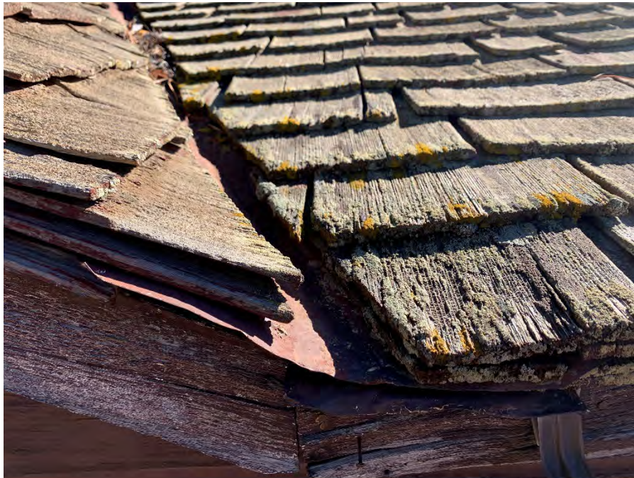
Figure 46: Detail view of sheet metal valley flashing.
