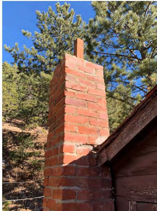
Figure 39: Brick chimney located to the northeast of the building.
