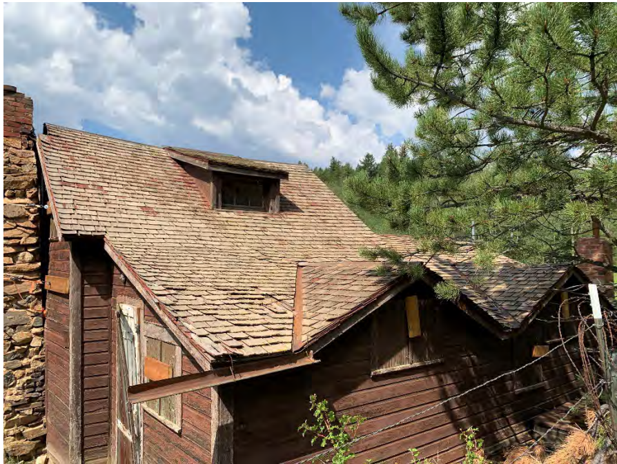
Figure 49: Half round gutter at the south end of the east elevation.
