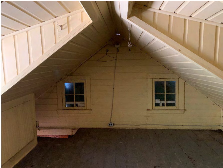
Figure 78: Overall view of finishes in the second floor bedroom.
