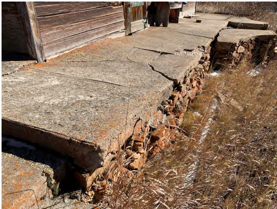
Figure 9: Patio / walkway along the west side of the building.
