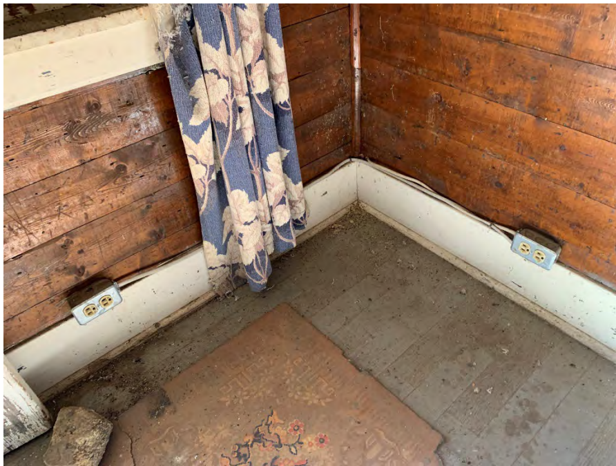
Figure 93: Painted wood base trim typical in the living room.
