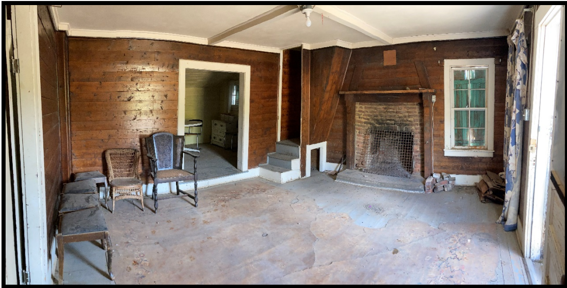
Tucker Cabin – living room overview after interior cleanup, steps to 2 nd floor are located to the left of the fireplace
