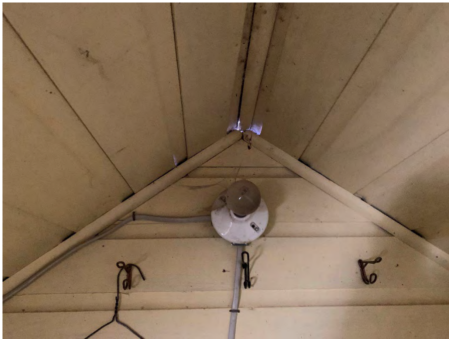
Figure 105: Light fixture located in the second floor bedroom.
