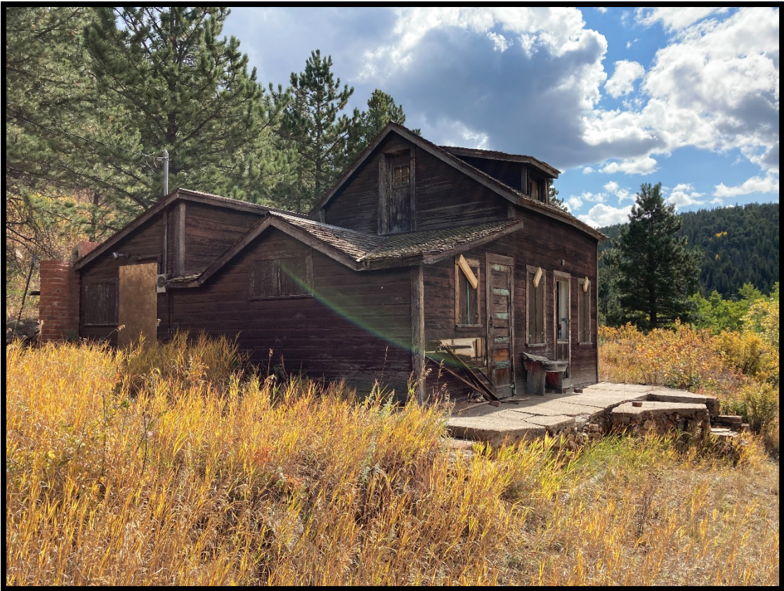
Tucker Cabin – southwest elevation
