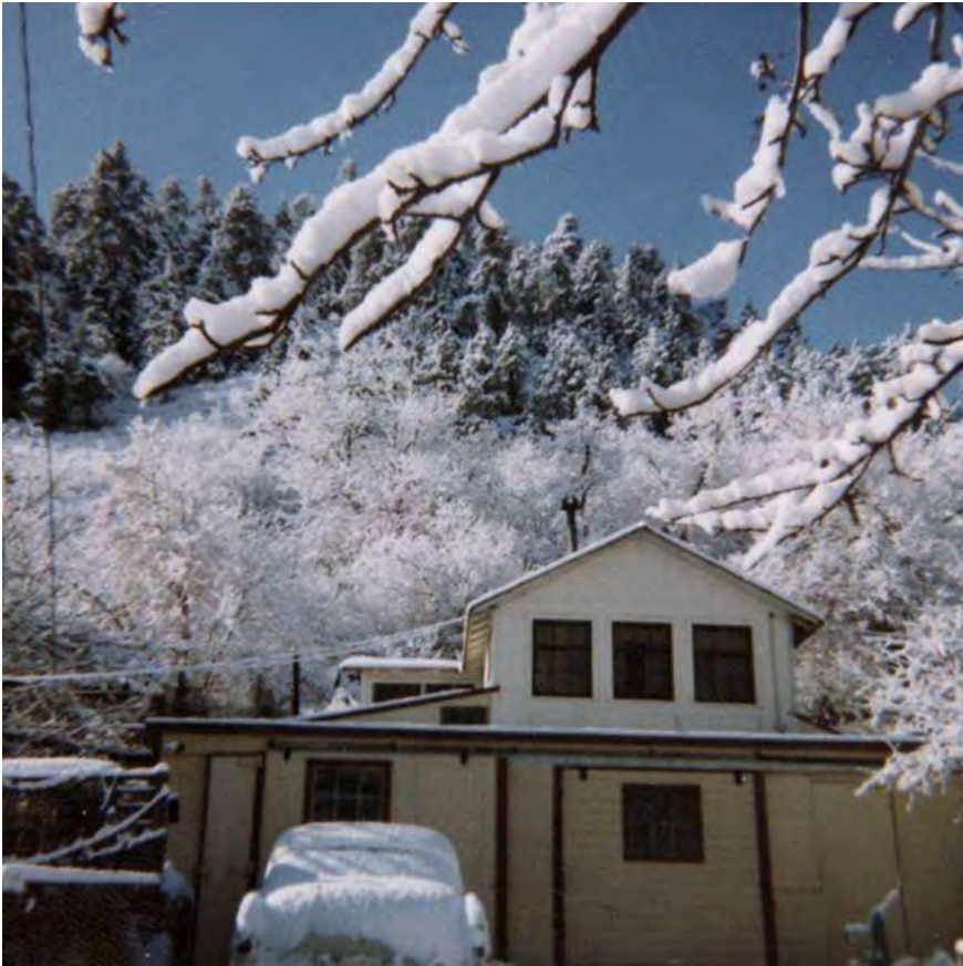
Garage and 2nd Story Apartment North Elevation 1964 Eldorado Springs: 59 Eldorado Springs Drive Carnegie Library Call Number 701-2-17
