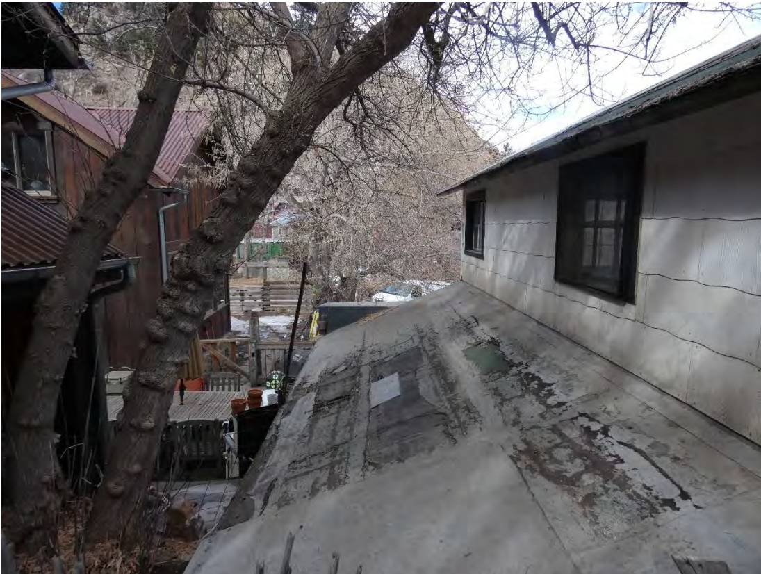
Garage and 2nd Story Apartment West Elevation February 2023
