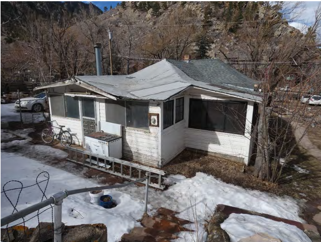
House South Elevation February 2023
