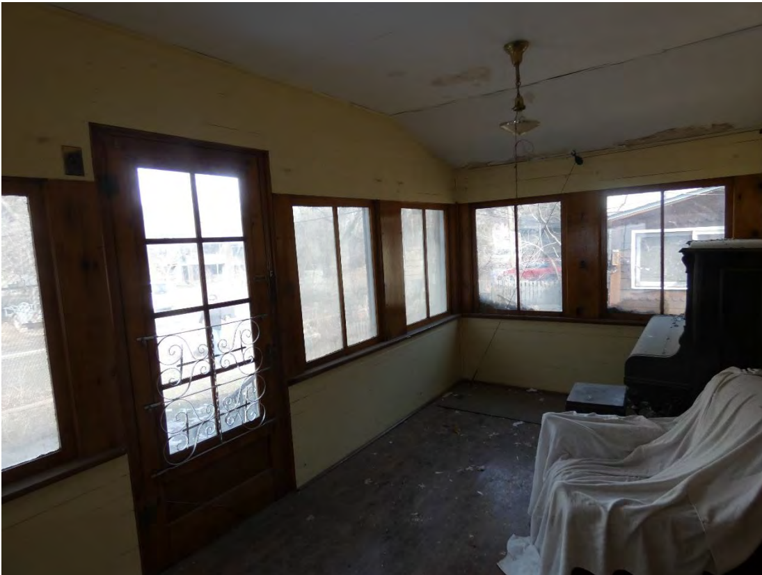
House Interior -North Closed in Porch February 2023
