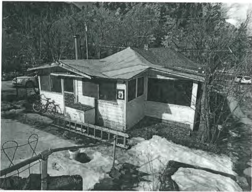
House South Elevation February 2023
