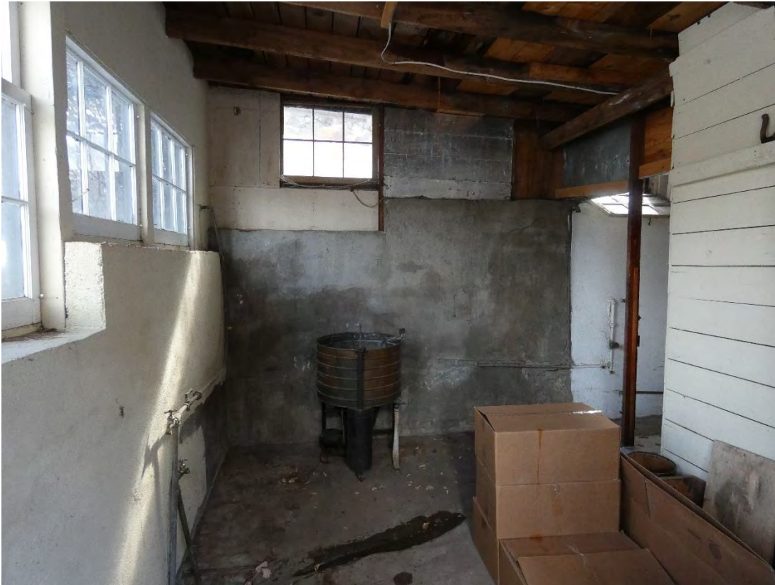
Interior-Far Left Room Garage and 2nd Story Apartment February 2023
