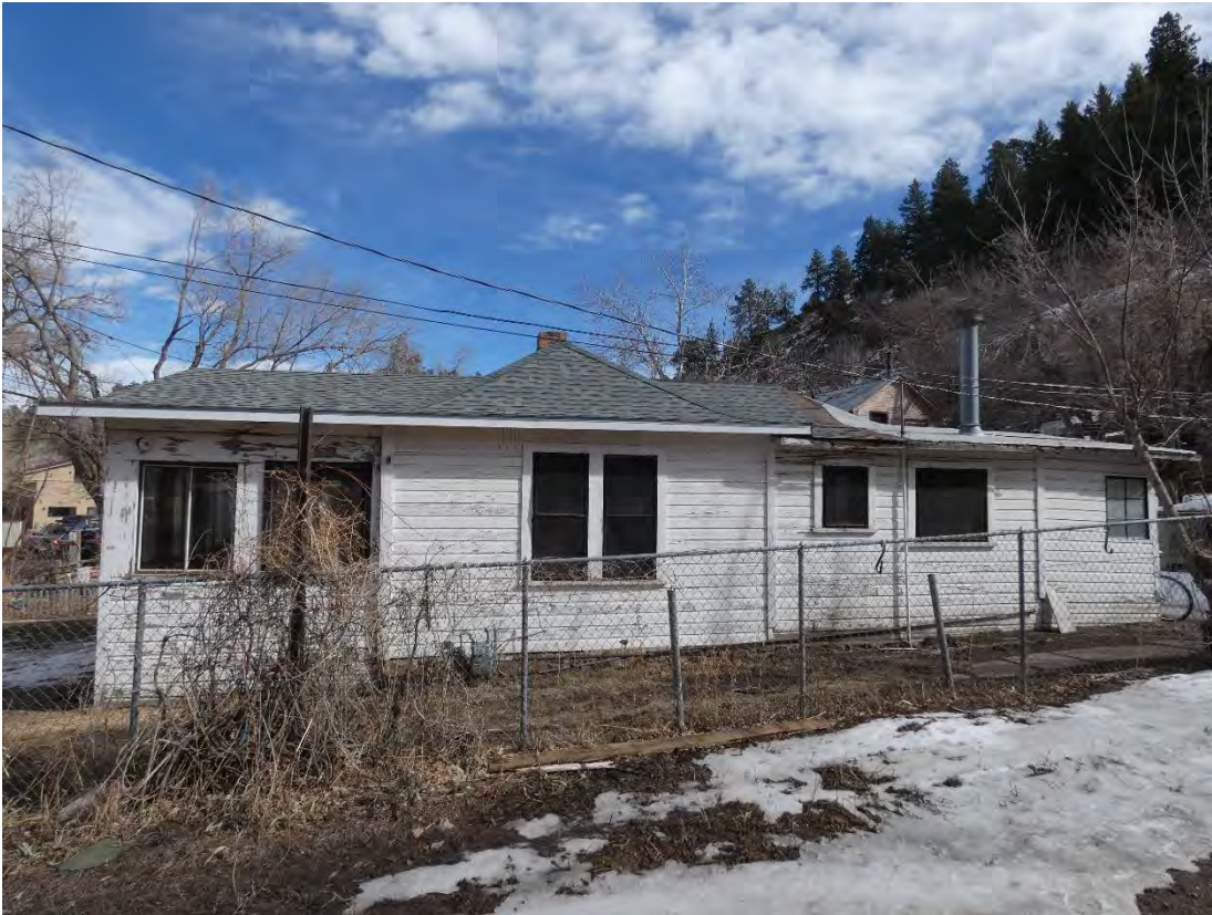
House West Elevation February 2023
