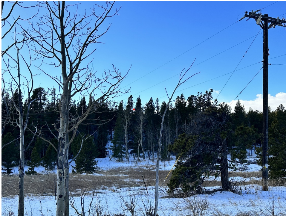
Photo #3, height pole flag is visible (marked with red dot):
