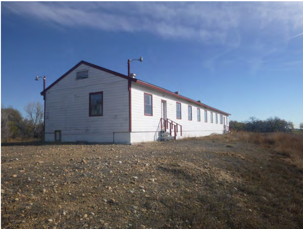
5BL5561 – Feature 1, bunkhouse, west and south elevations, view to the northeast. Photo Number: D3.0295 Date: 10.28.15
