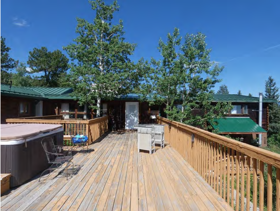
Lodge East Elevation July 2023
