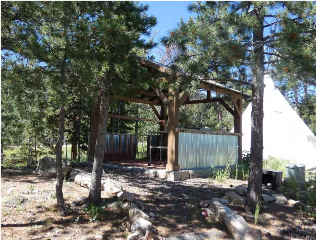
Gazebo Northeast Elevation July 2023
