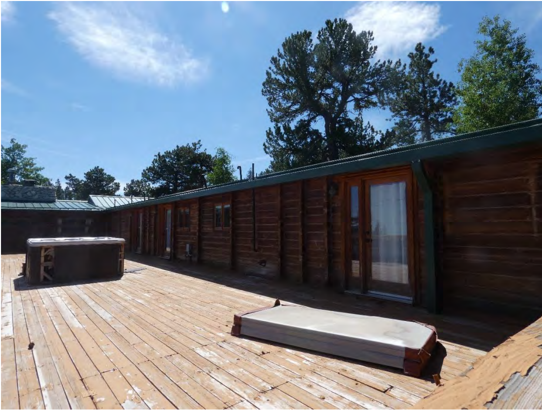
Lodge Northwest Elevation July 2023
