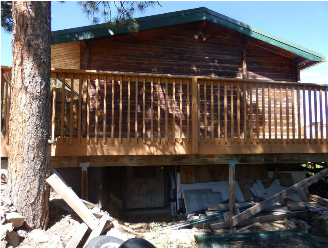
Lodge East Elevation July 2023
