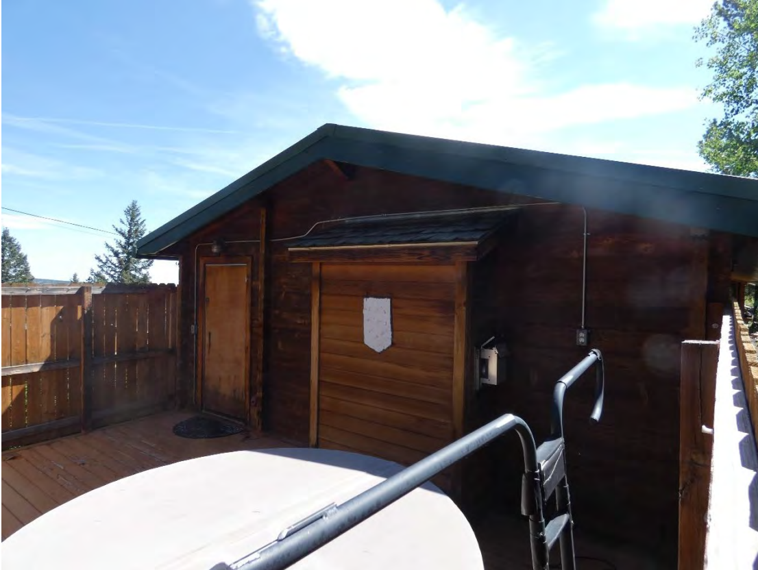
Lodge West Elevation July 2023
