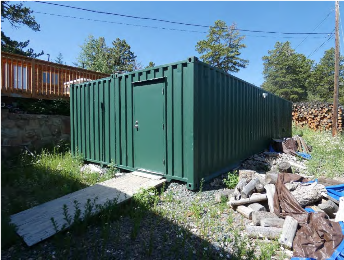
Shipping Container Southeast Elevation July 2023
