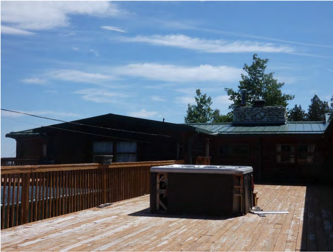
Lodge West Elevation July 2023
