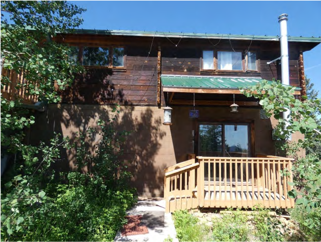
Lodge East Elevation July 2023
