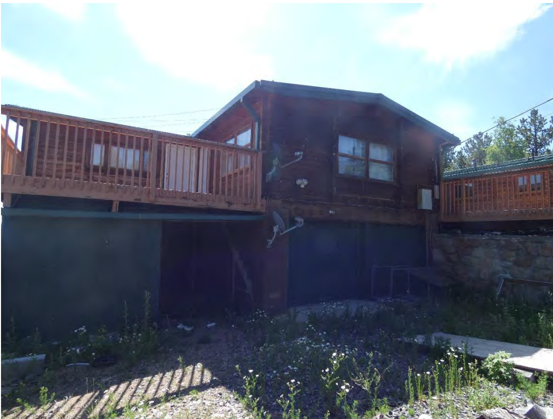
Lodge West Elevation July 2023
