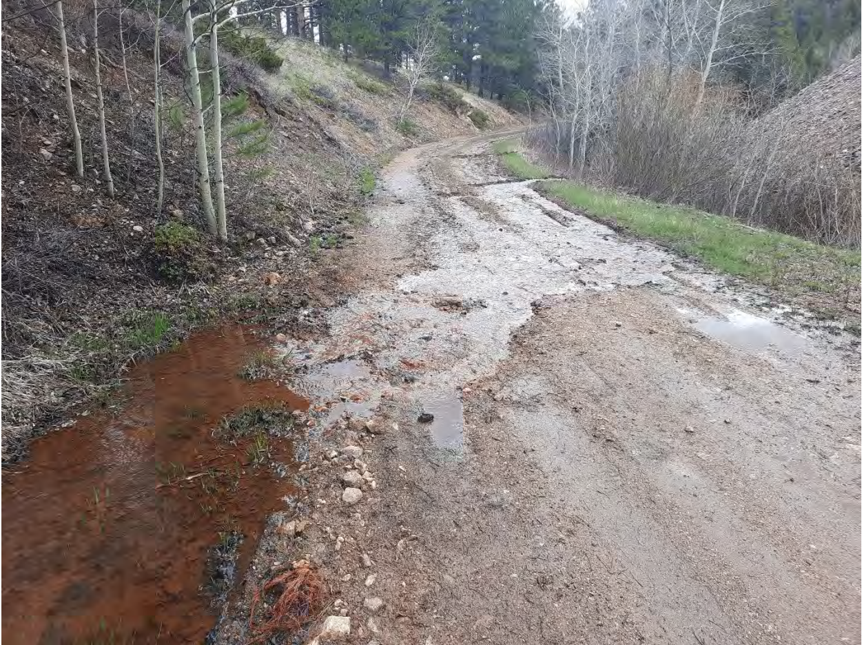
Figure 10. Sherwood Creek and additional north slope seepage running on access road before entering impacted historic creek channel.
