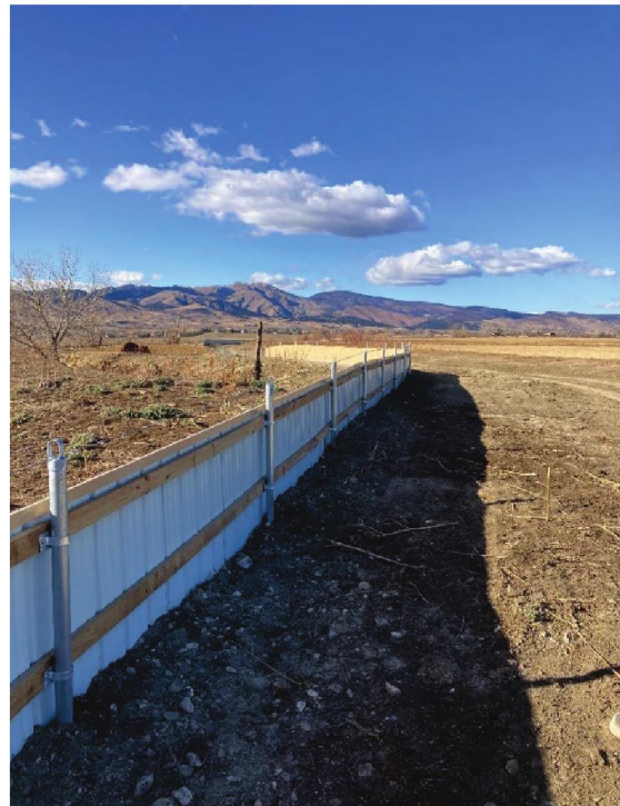
Figure 1. Metal barrier prairie dog fence. Fence Section A in Site Plan.
