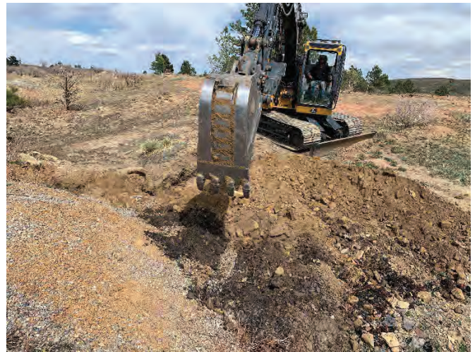
PHOTOGRAPH 28 Test Pit 5 in the OSM reclamation area.
