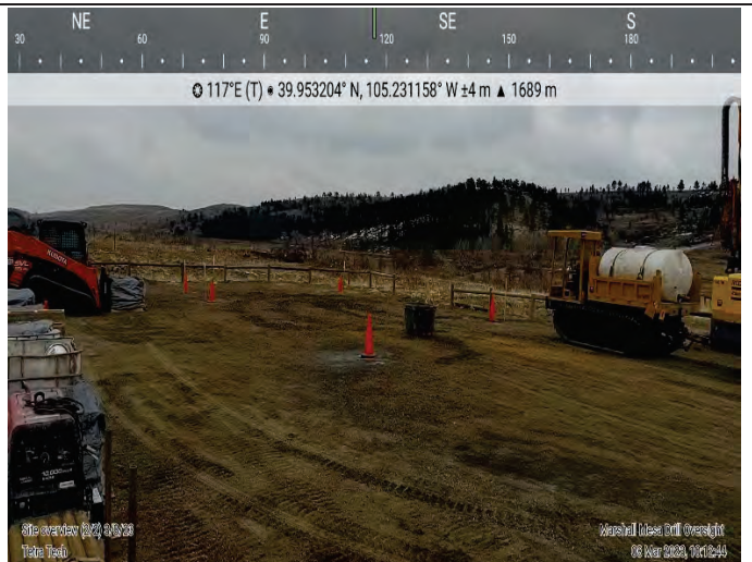
PHOTOGRAPH 18 03-08-2023 Site overview looking southeast from parking lot
