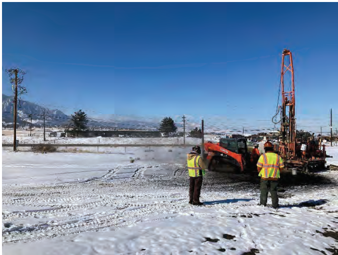
PHOTOGRAPH 9 02-24-2022 MM-06 Drilling through coal.
