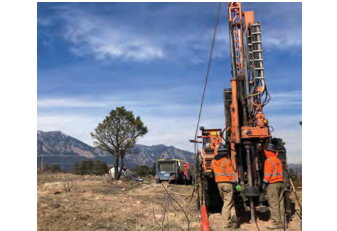
PHOTOGRAPH 24 Drilling MM-36, view to the west.
