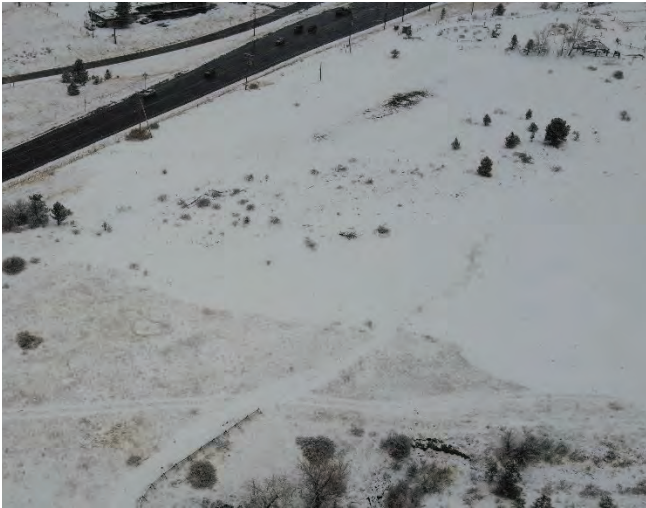
PHOTOGRAPH 7 03-06-2022 UAV snowmelt looking Northwest.
