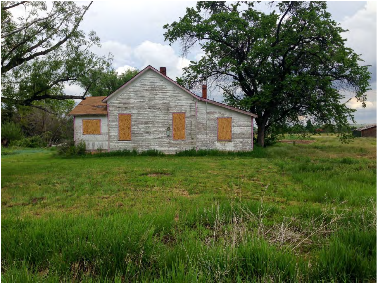
The old house that was demolished. This house presented a danger to the neighborhood because of chemical (e.g., asbestos) and biological hazards. Children could have easily broken into the house and exposed themselves to these hazards.
