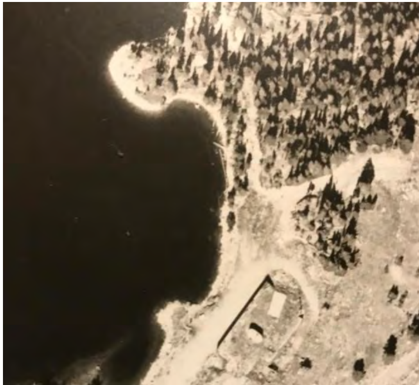
Underground house and maintenance road, circa early 90's
